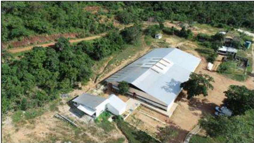
Figure 5.3 – Cerrado Gold Core Logging Area and Office
