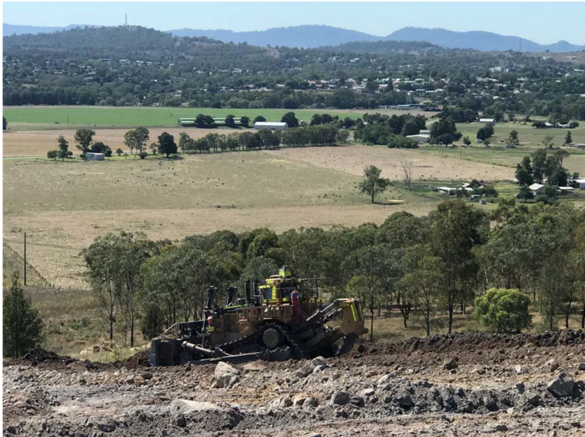
Plate 2: Eastern Out of Pit Emplacement Rehabilitation
