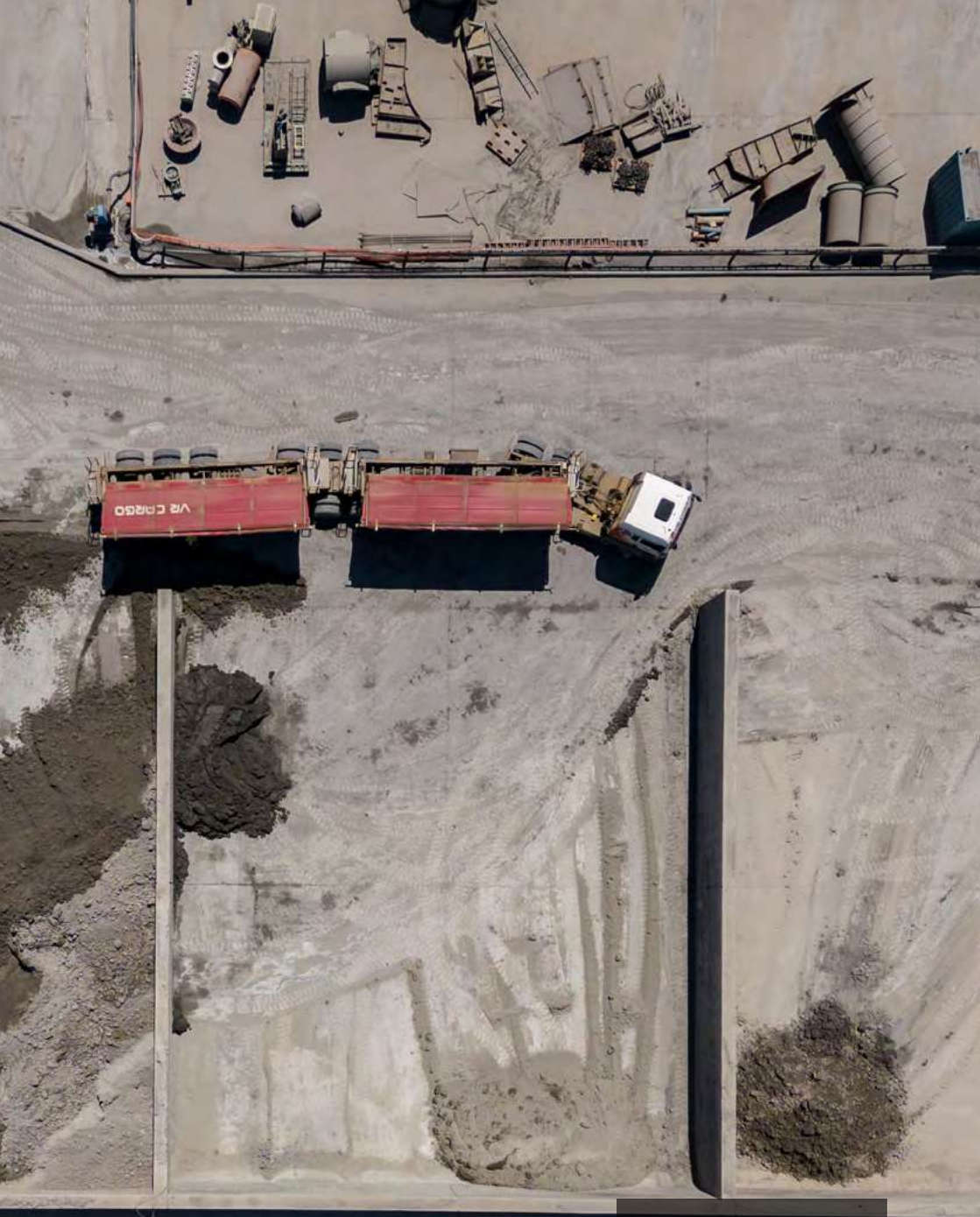
Concentrate storage bays at Zondereinde metallurgical complex
