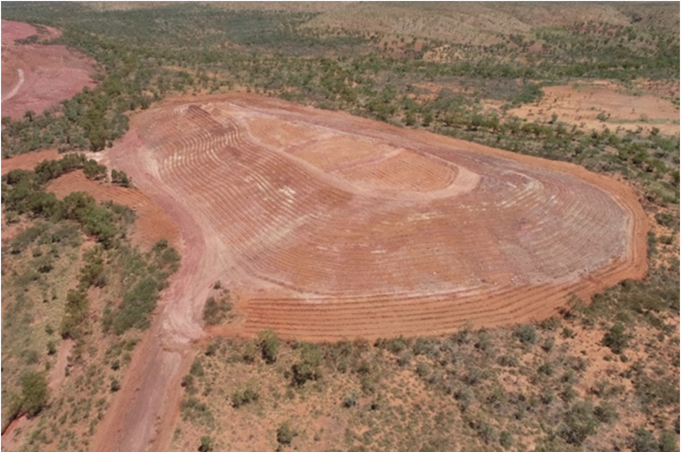
Figure 4: Profiling, topsoil spread, drainage and cross-rip completed.
