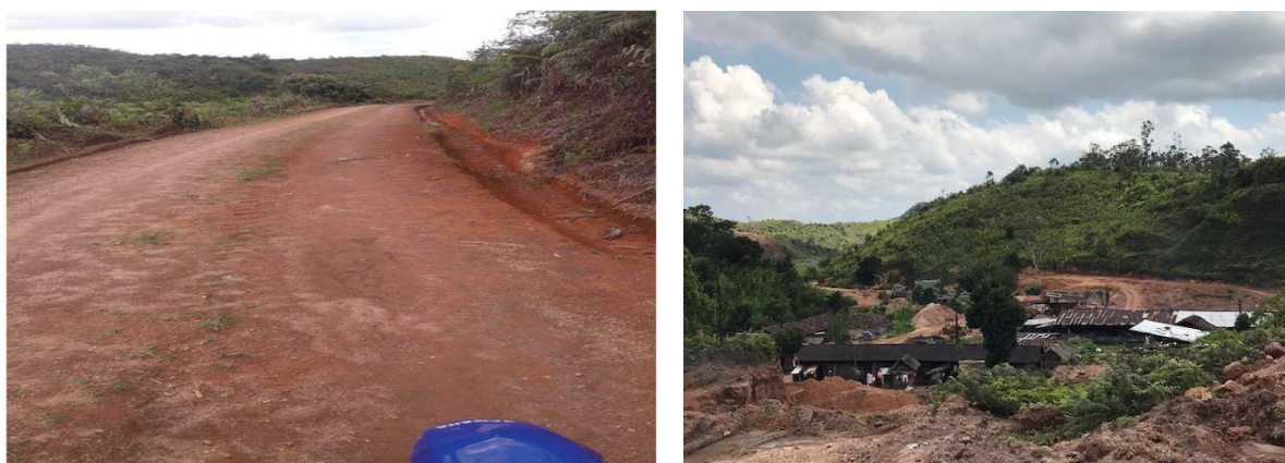
Figure 33 - Upgraded approach road to Sahamamy and view of existing plant site
