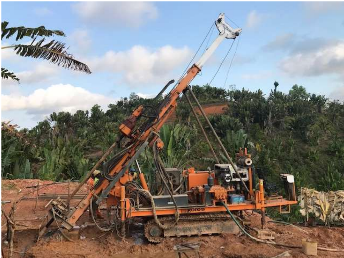
Figure 26 - TG's new track-mounted diamond rig on site at Vatomina
