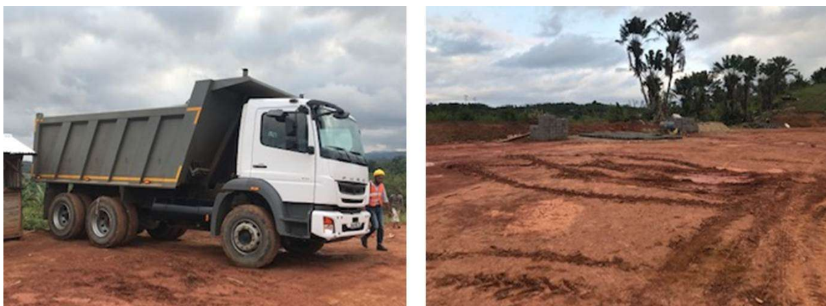
Figure 28 - Earth moving equipment on site and site clearance well advanced
