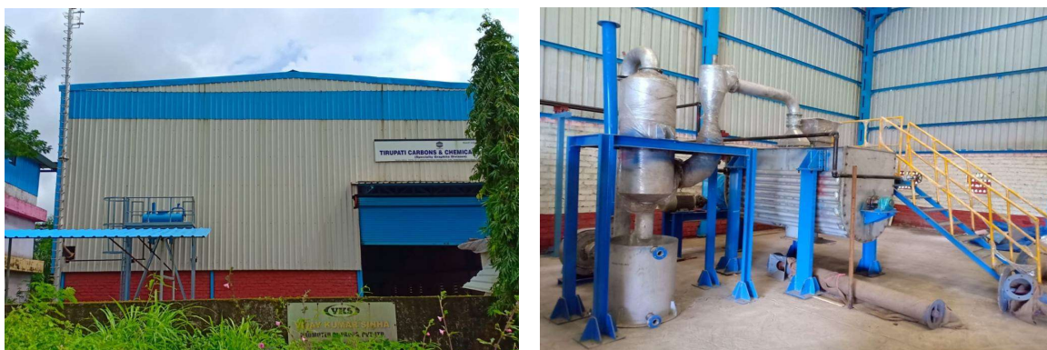
Figure 39 - 1,200tpa fire retardant facility near Mumbai India
