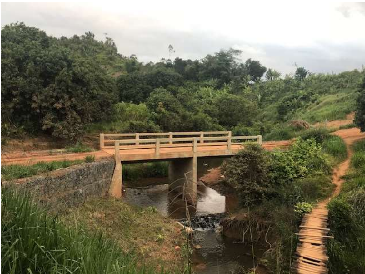
Figure 32 - New bridge on the Vatovina permit
