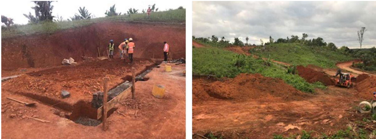
Figure 29 - Foundations for warehouse and site clearance for processing plant
