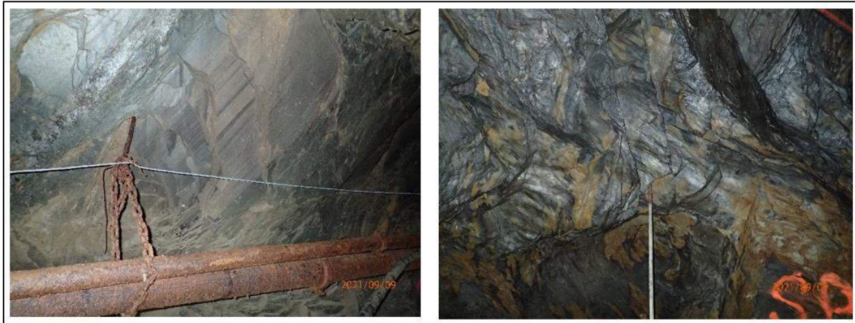
Figure 7-6: D2 and D3 Fold Plunges
