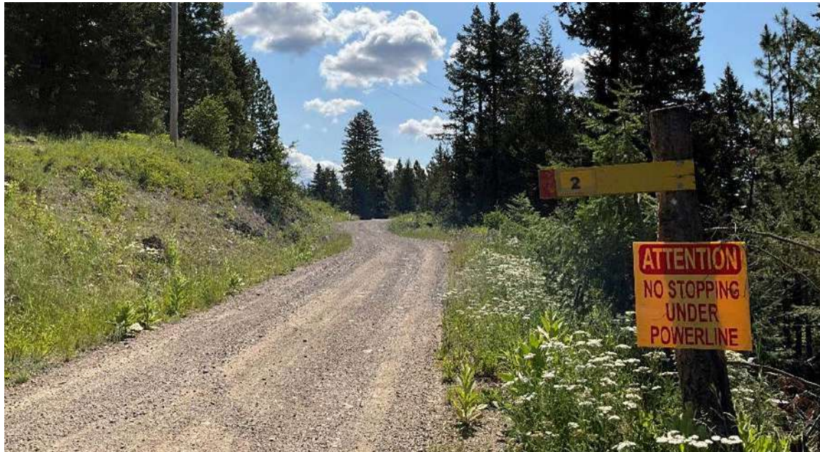
FIGURE 5.8 TYPICAL ROAD AREA OF SOUTH SHOVELNOSE ROAD
