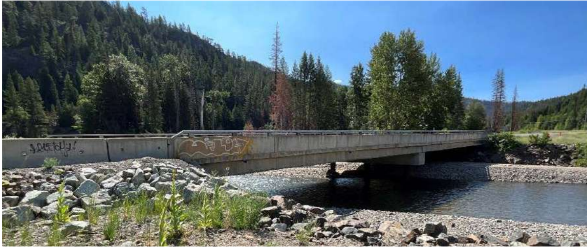
FIGURE 5.5 BRIDGE NO.1 ON THE COLDWATER ROAD
