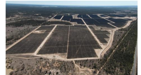
Completed Edenvale Solar Park in Sep. 2023
