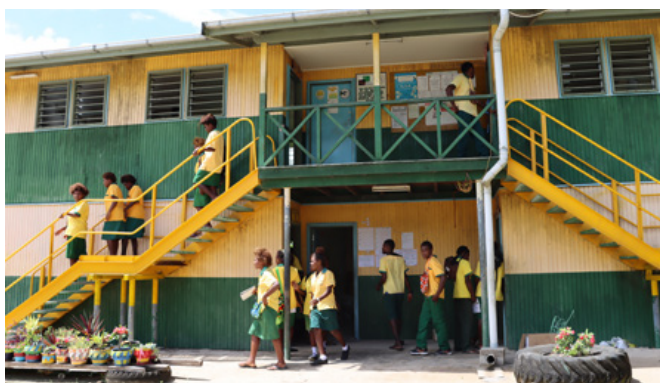
New metal stairs for the local school double classroom.
