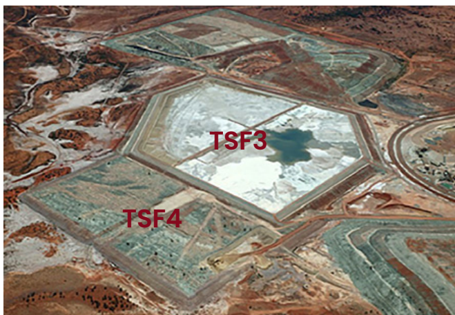
Gwalia mine's TSFs 3 and 4.
