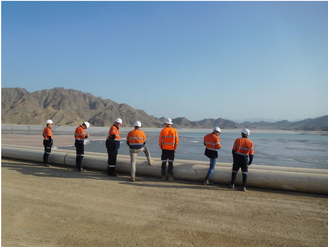
Photo 18.1: TSF No. 2, Viewed from the North
