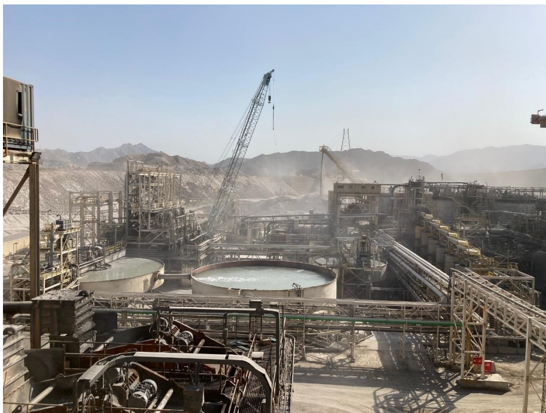
Photo 17.1: Sukari Process Plant
