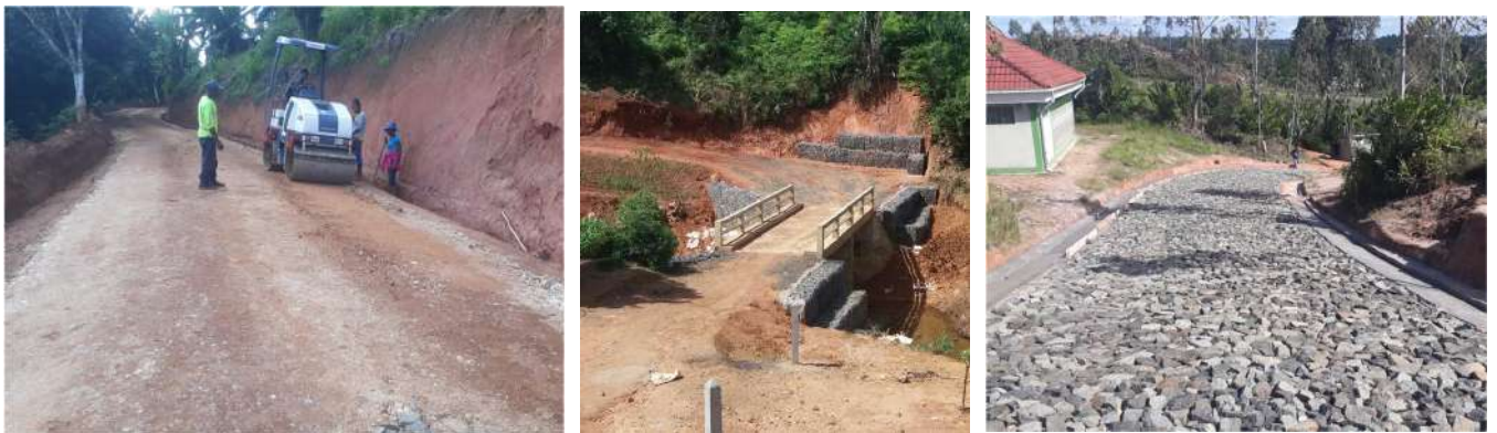
Fig. 13: Self constructed 11m long bridge, internal roads
