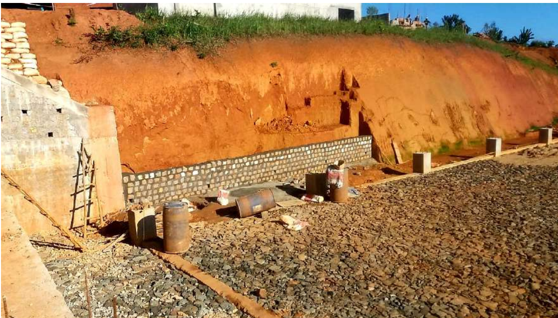
Fig.: 6000TPA plant under construction
