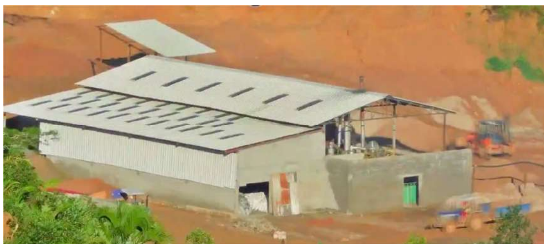
Fig.: 3000 TPA Processing Plant
