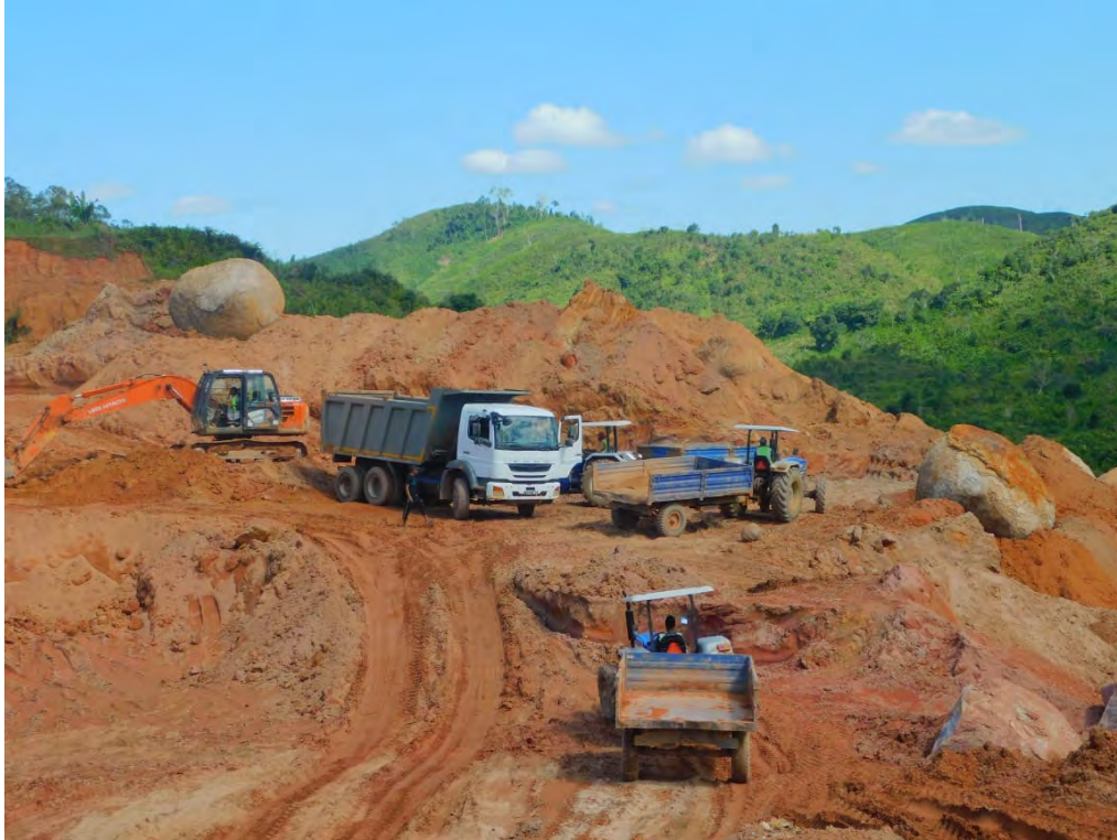
Figure 6-4: Hauling machinery in Sahamamy
