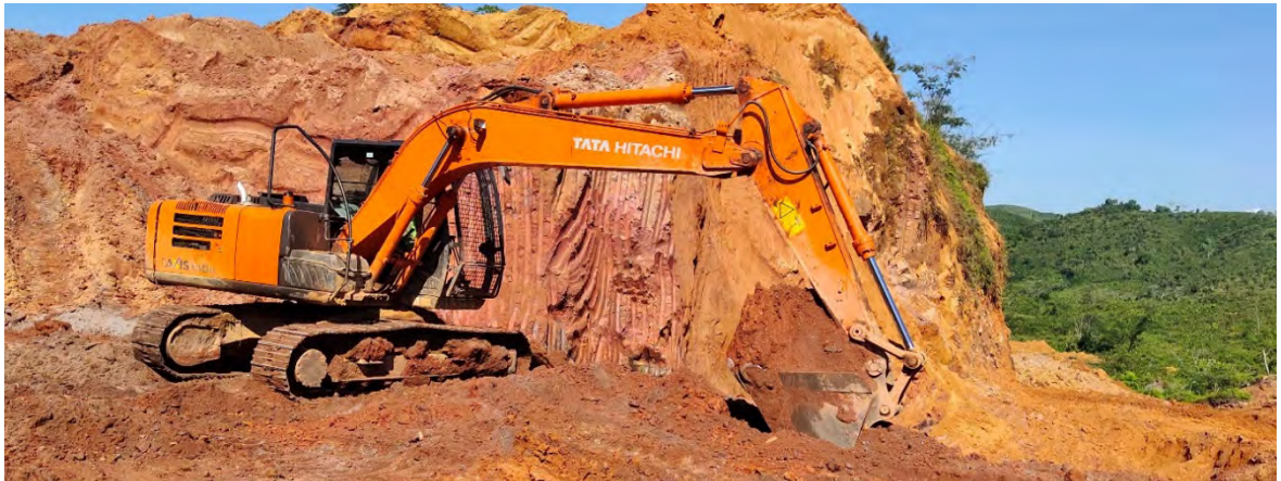
Figure 6-3: Excavator in operation in mining area B
