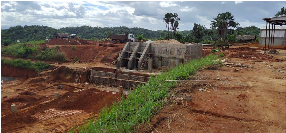
Figure 7-6: Vatomina: truck unloading point; under construction
