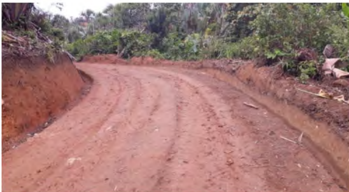
Figure 8-4: Dedicated approach road to Sahamamy was widened (to 6m) and strengthened
