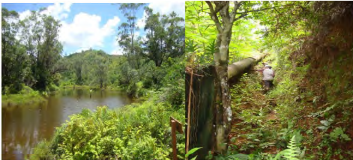
Figure 8-7: Reservoir and pipeline for an old hydro power plant (now non-operational) at Sahamamy; Tirupati proposes to revive the hydro power plant in due course
