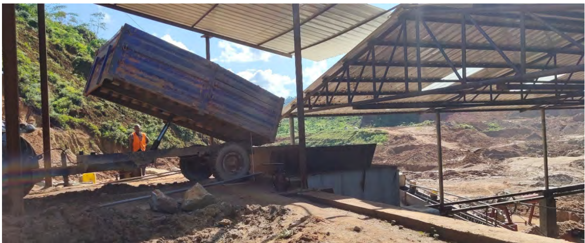
Figure 6-5: Dumping of ore at processing plant hopper
