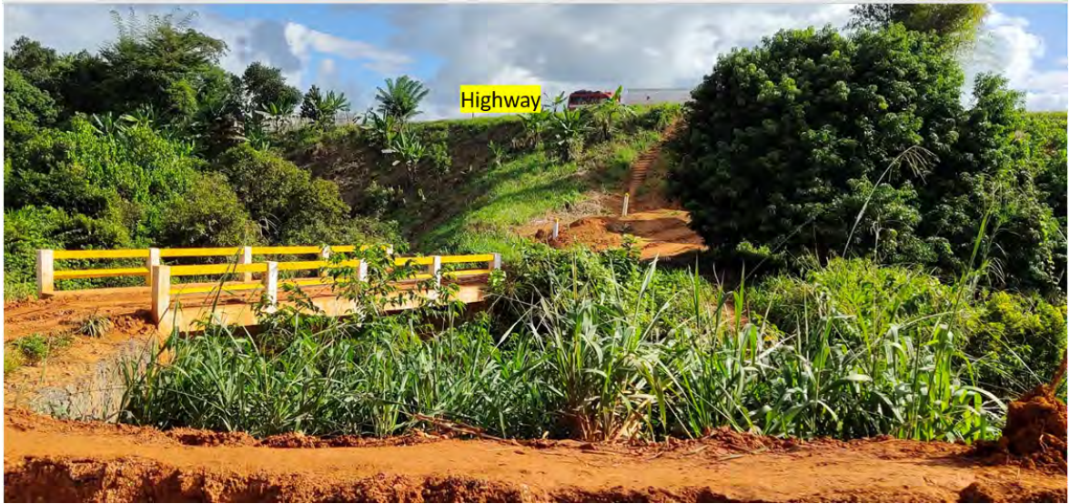
Figure 8-9: Newly constructed bridge connecting Vatomina site to the National Highway
