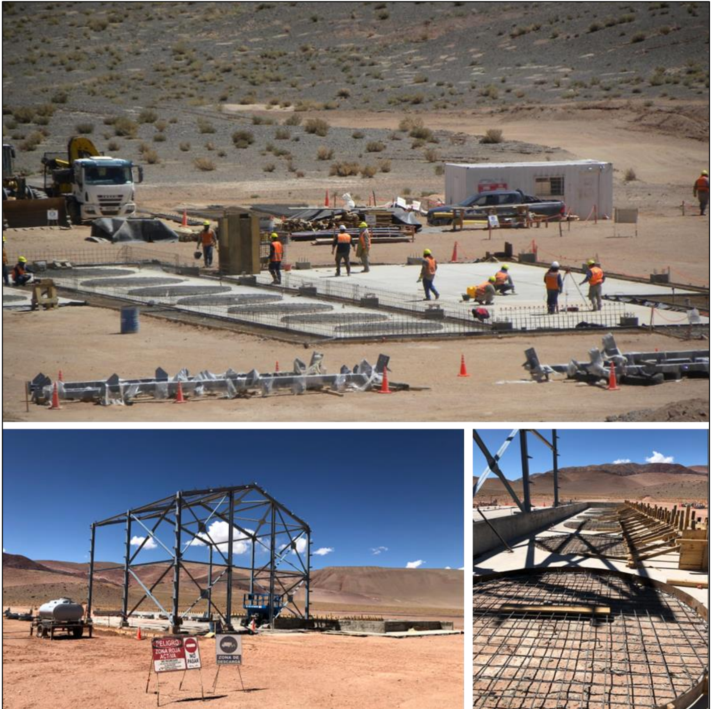
Figure 13-11: Photographic Record of Pilot Plant Construction
