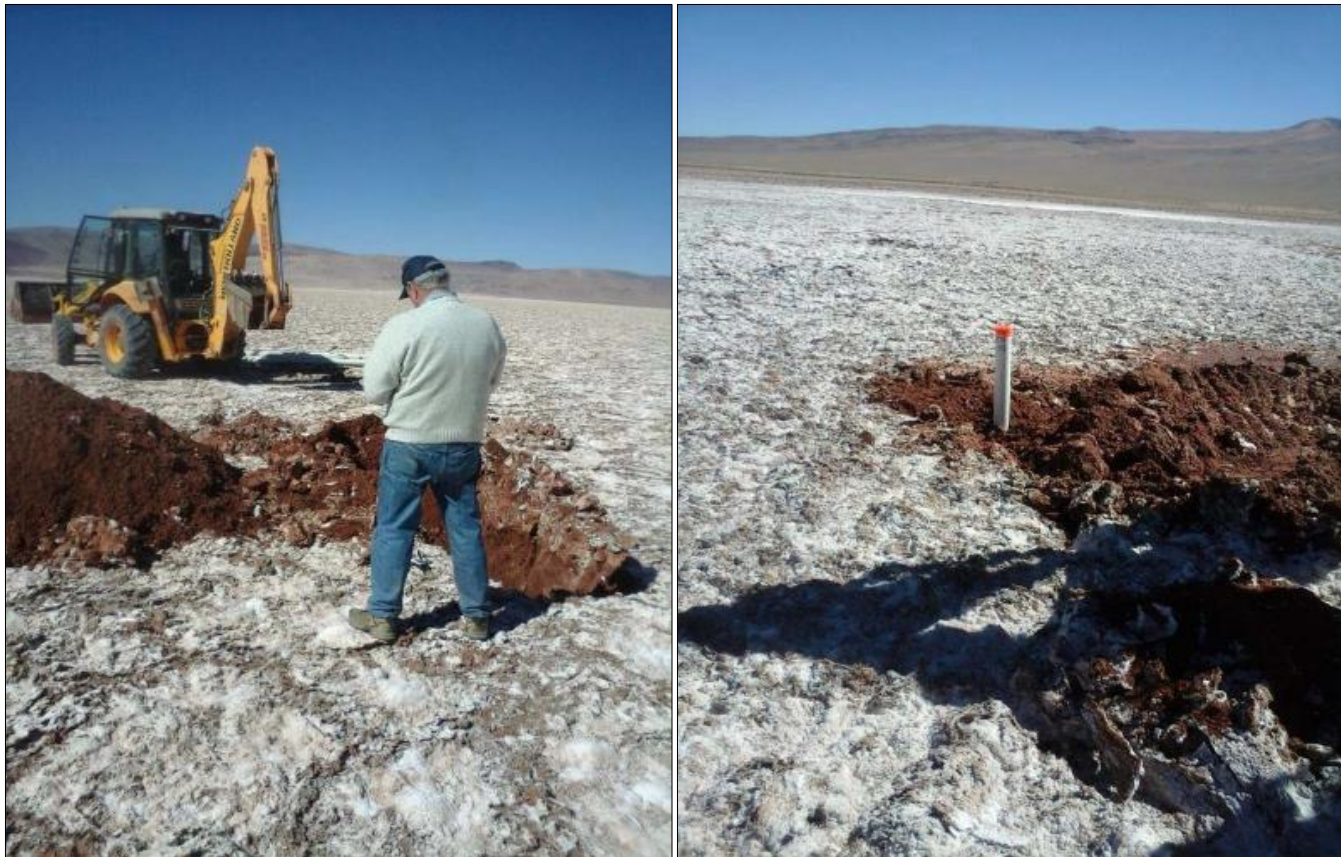
Figure 6-2: 2014 Trench (left) and PVC Tube Installed After Trenching (Right)
