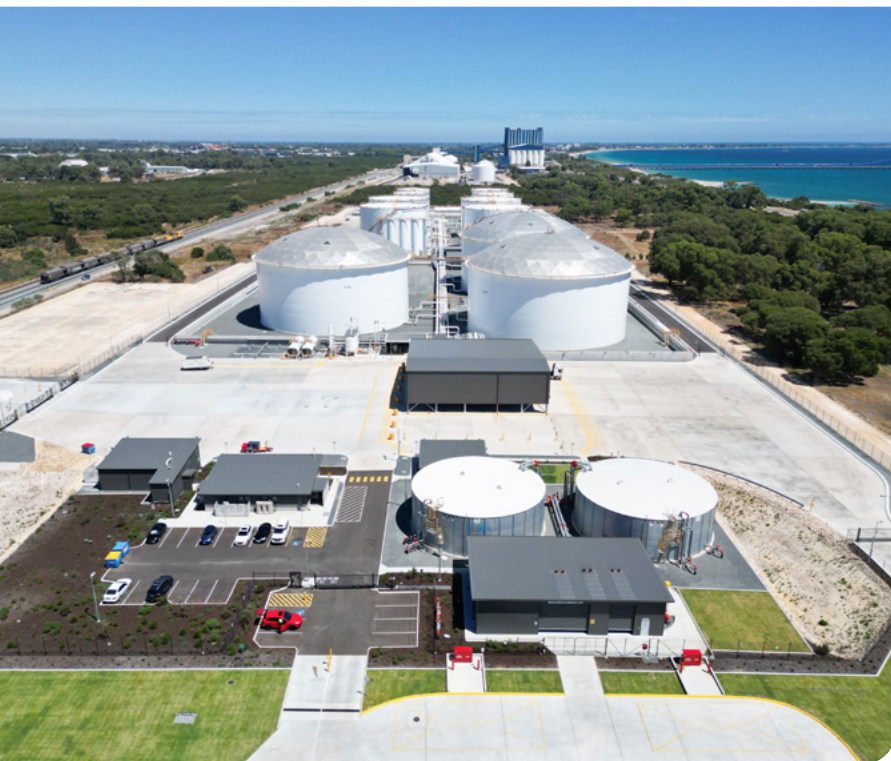
↑ The newly-commissioned 200,000cbm Impala Terminals energy import, storage and distribution terminal in Kwinana, Australia.
