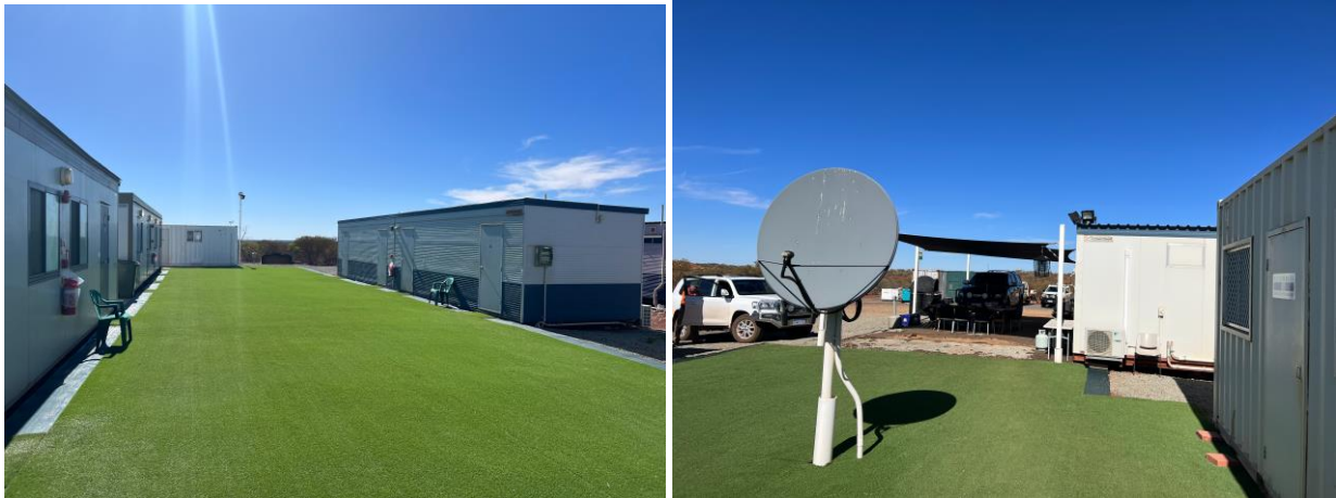
Figure 5-2 Exploration Camp Facilities
