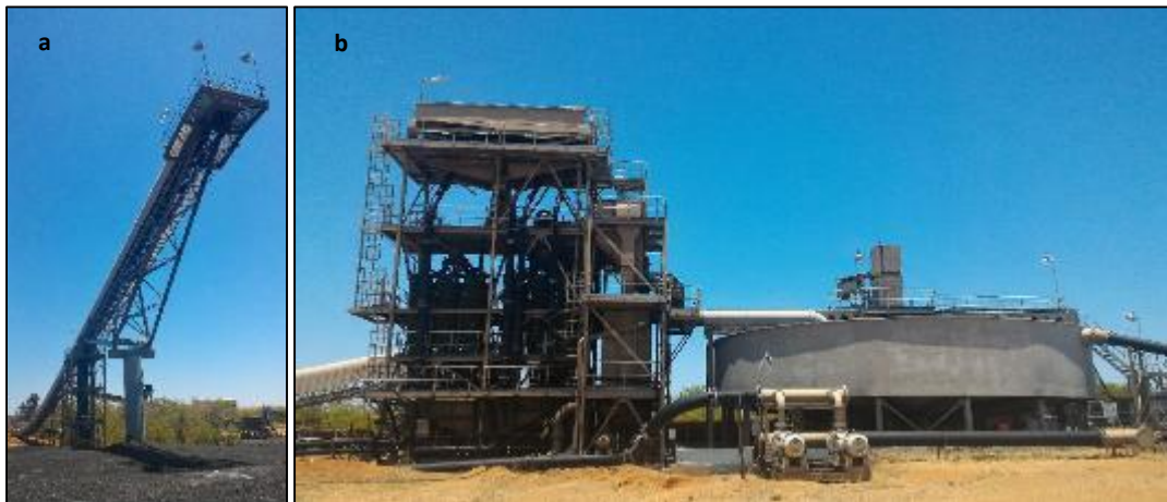
Figure 8.3.2: (a) Existing stockpile facility (lined, with rathole) (b) Cyclone and thickener module
