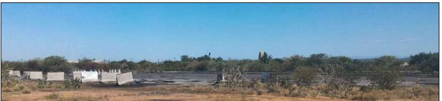
Figure 8.2.5: Rail siding stockpile area in Musina with concrete base
