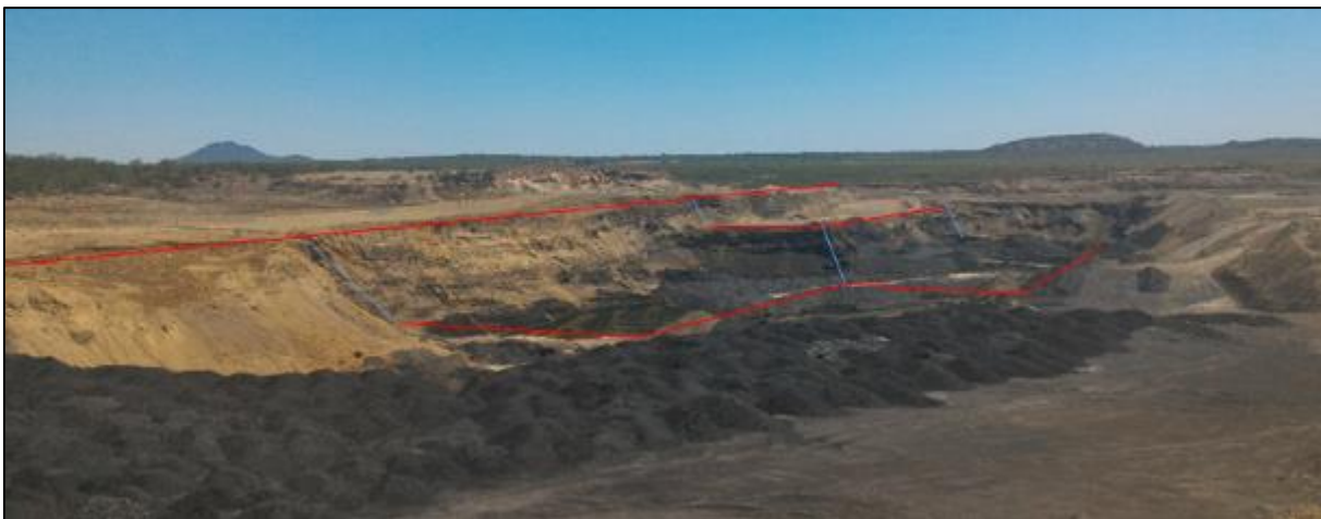
Figure 8.2.3: Existing opencast with open benches indicated by red lines, and carbonaceous backfilling in foreground
