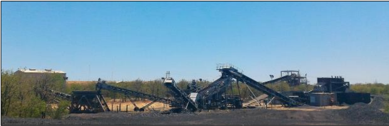
Figure 8.3.1: Existing Coal processing plant module
