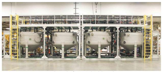
Figure 17.4: Chemical Softening with Solid-Liquid Separation
