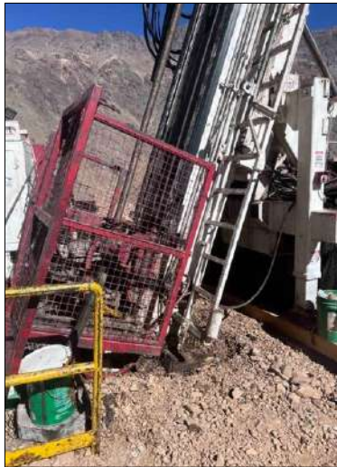
Figure 12.2: Drill Hole CMV-012b, Drilling
