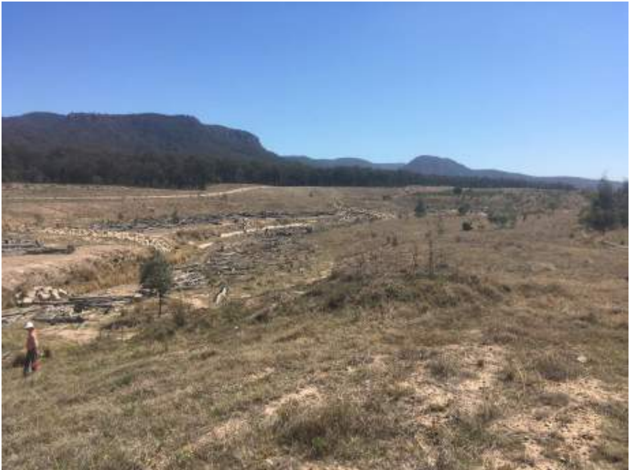
Plate 19: North Wambo Creek Diversion during 2018 at site 26R
