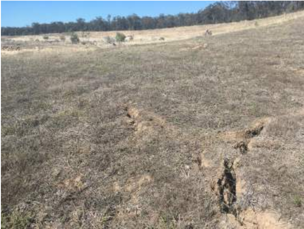
Plate 27: Subsidence cracks near rehabilitation monitoring site 28R
