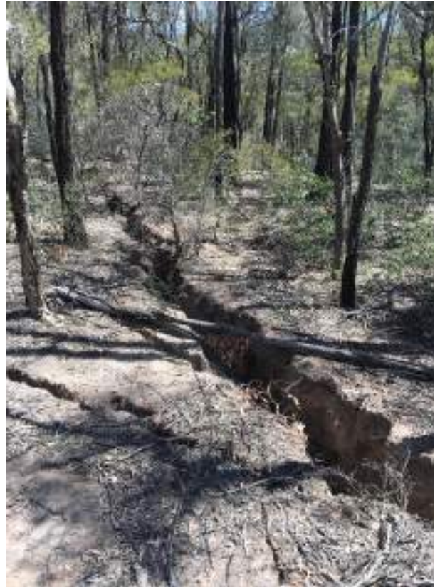
Plate 26: Large subsidence cracks near flora monitoring site V11-B1
