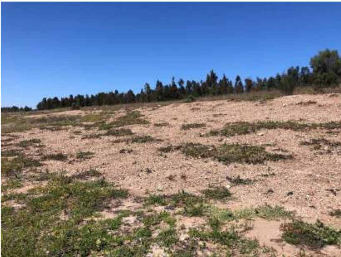
Photograph 44: Large area of erosion/bare soil at failed pasture rehabilitation near site 33R (exceeding completion criteria)
