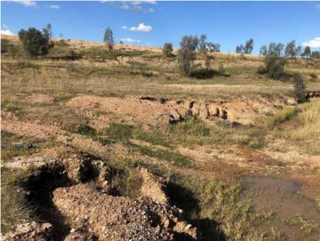
Photograph 21: Gully erosion within the North Wambo Creek Diversion (near site 23R) in 2020
