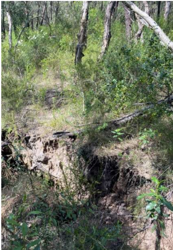
Photograph 36: Large subsidence cracks near flora monitoring site V11-B1 (in 2022)
