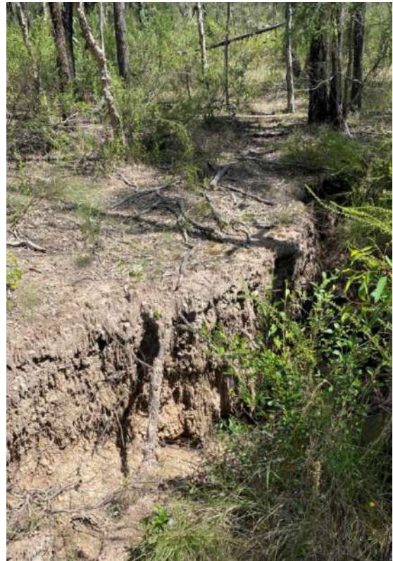
Photograph 37: Large subsidence cracks near flora monitoring site V11-B1 (in 2022)
