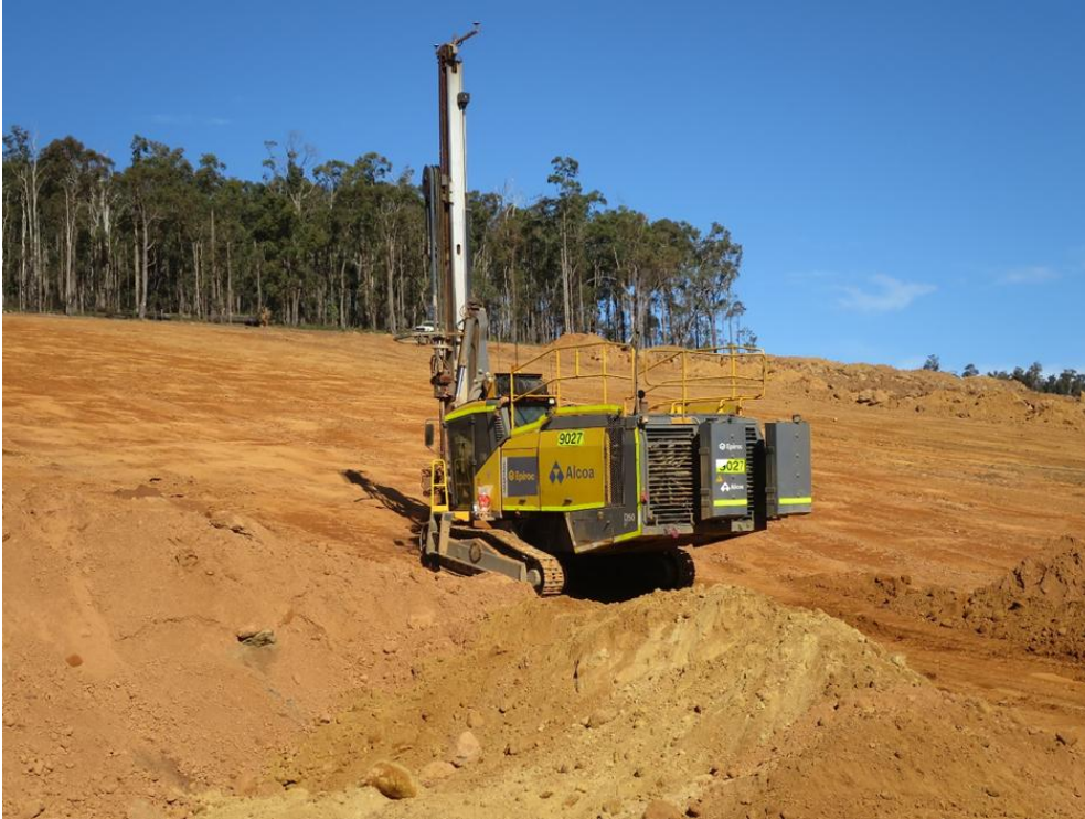
Figure 13-12: Blasthole Drill Working on Hardcap (SLR, 2021)
