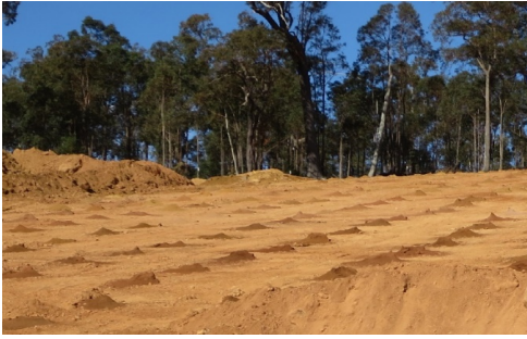
Blastholes on Hardcap after sheeting with low grade
