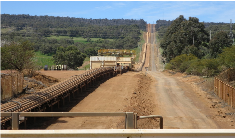
Figure 13-6: Covered Conveyor (SLR, 2021)
