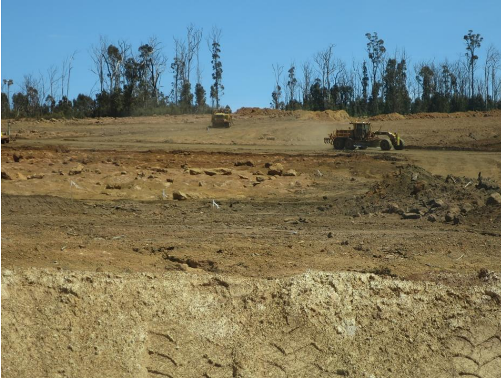
Figure 13-2: Topsoil Removal (Background), Blasting of Hardcap and Marking of Ore (foreground) (SLR, 2021)
