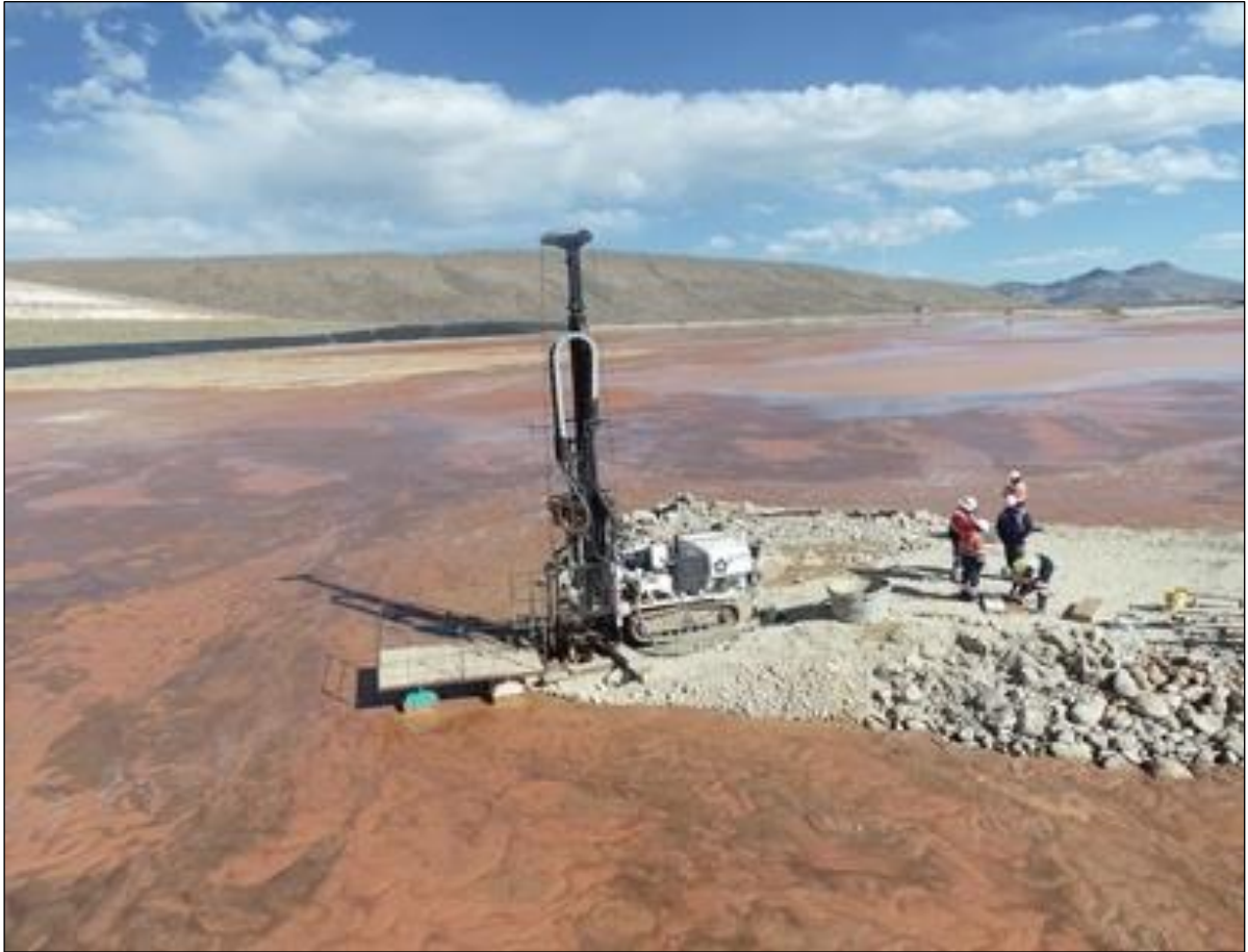
Figure 10-2: Sonic Drilling within the FDF
