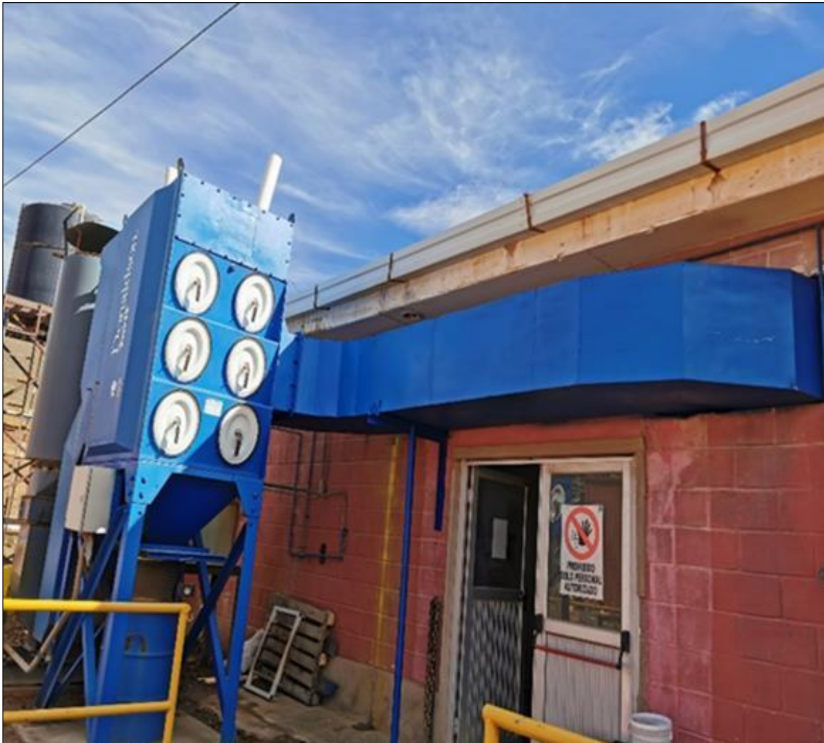
Figure 11-3: Donaldson Lead Collector
