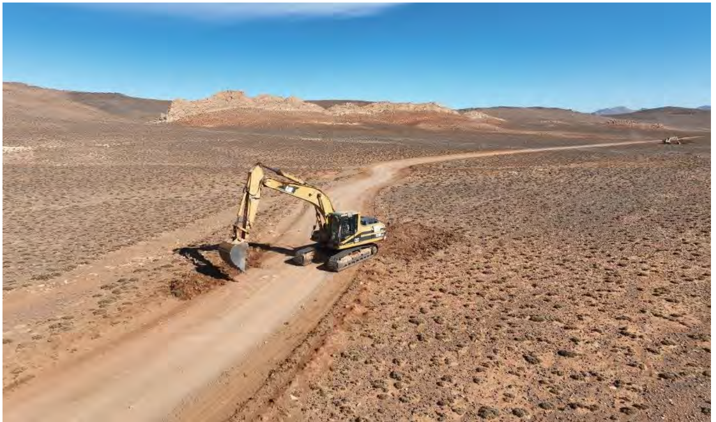
Figure 7 - Repair and Widening of Road Section Between Two Rural Villages
