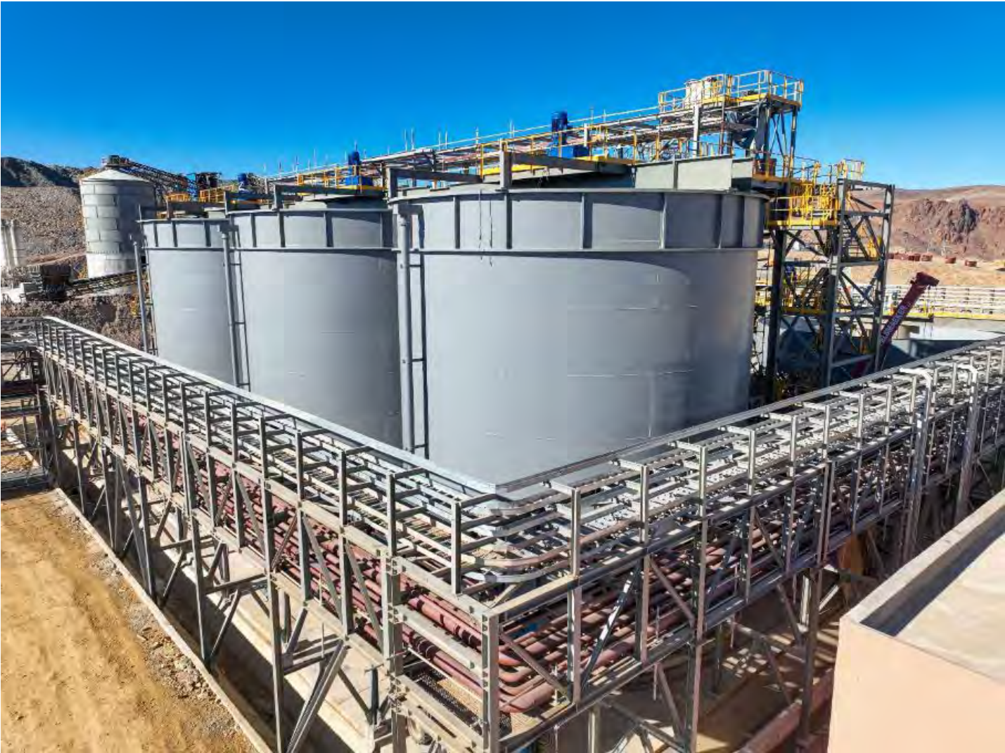
Figure 2 - Completion of Leaching Tanks
