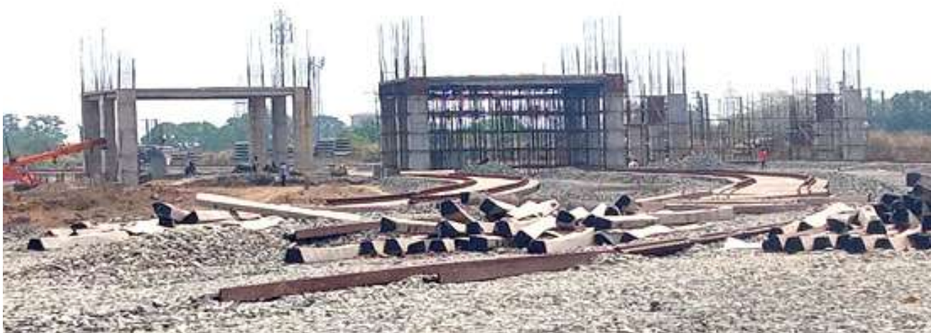
2.5 Mtpa Patherdih NLW WASHERY UNDER CONSTRUCTION
