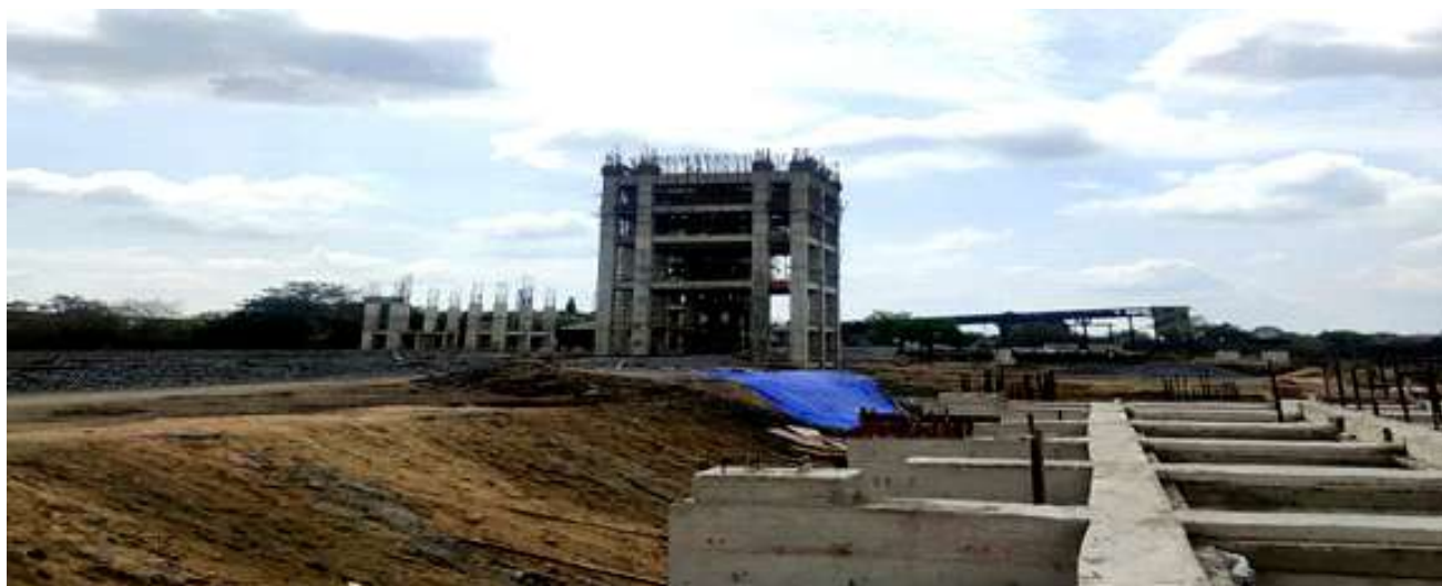
2.0 MTPA BHOJUDIH NLW WASHERY UNDER CONSTRUCTION
