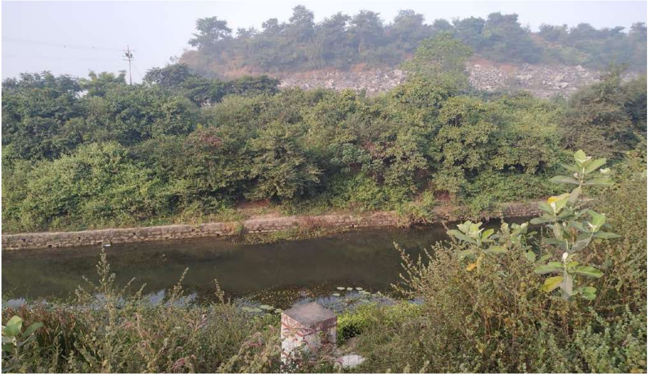
Stone Pitching along the water body
