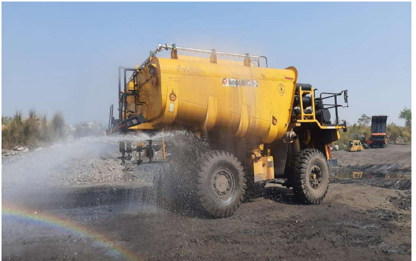
Water Sprinkling on Haul roads through Mist type water tanker
