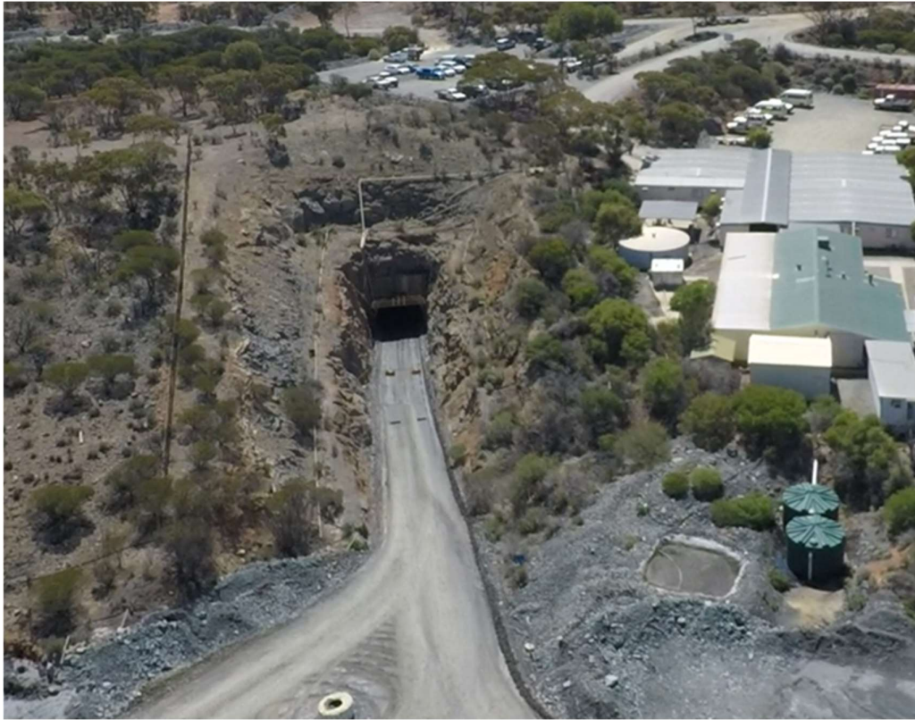
Figure 16-6 West decline portal and surface layout
