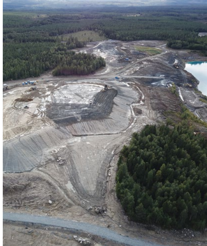
Reclamation work at the closed Rävildmyr mine.
