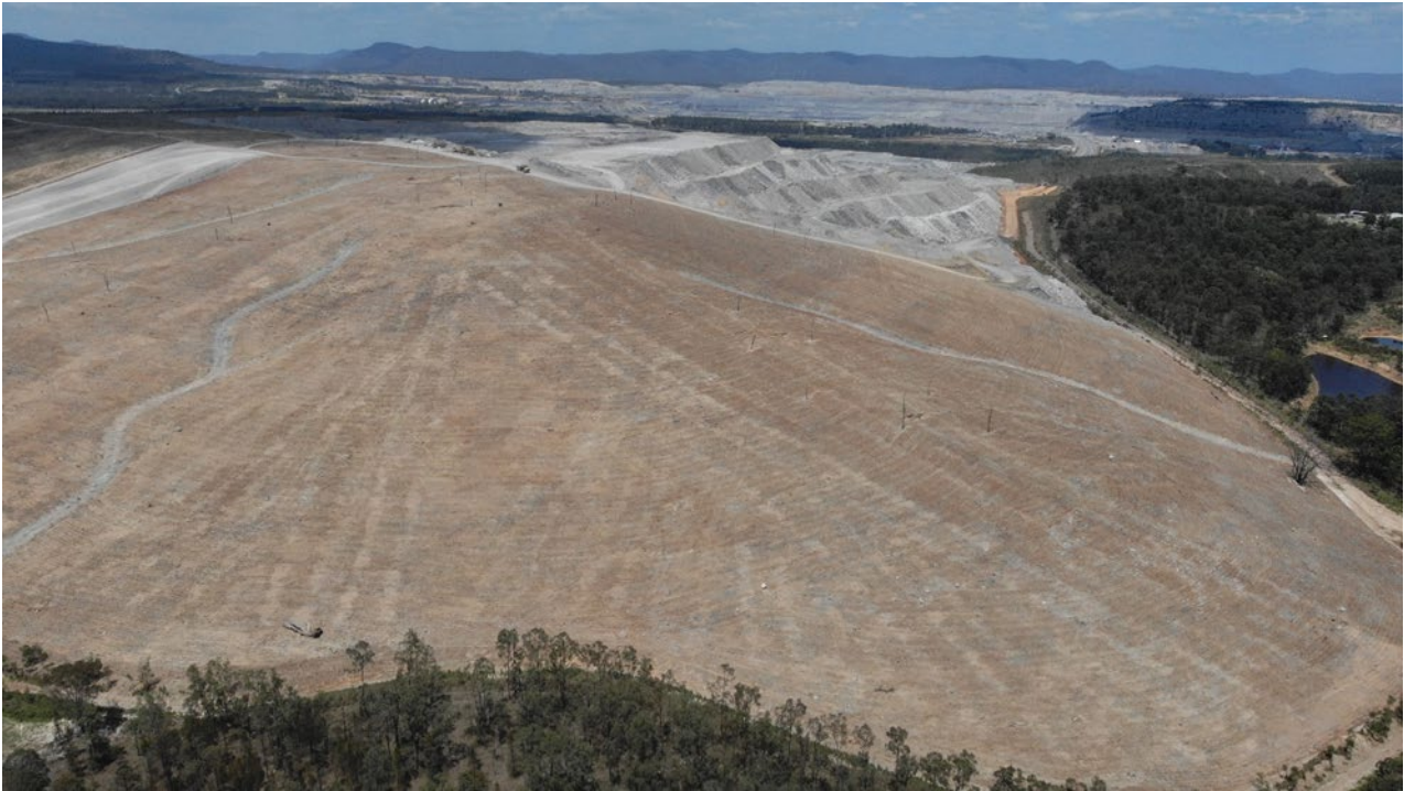
Photo 8.1 Rehabilitation completed in 2023 at the Eastern Emplacement Area
