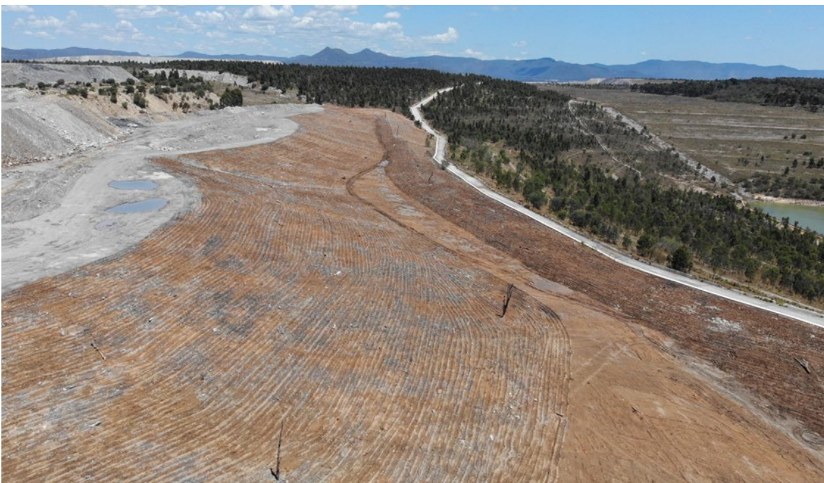
Photo 8.2 Deep ripping of topsoil in progress at the East Pit Emplacement in 2023
