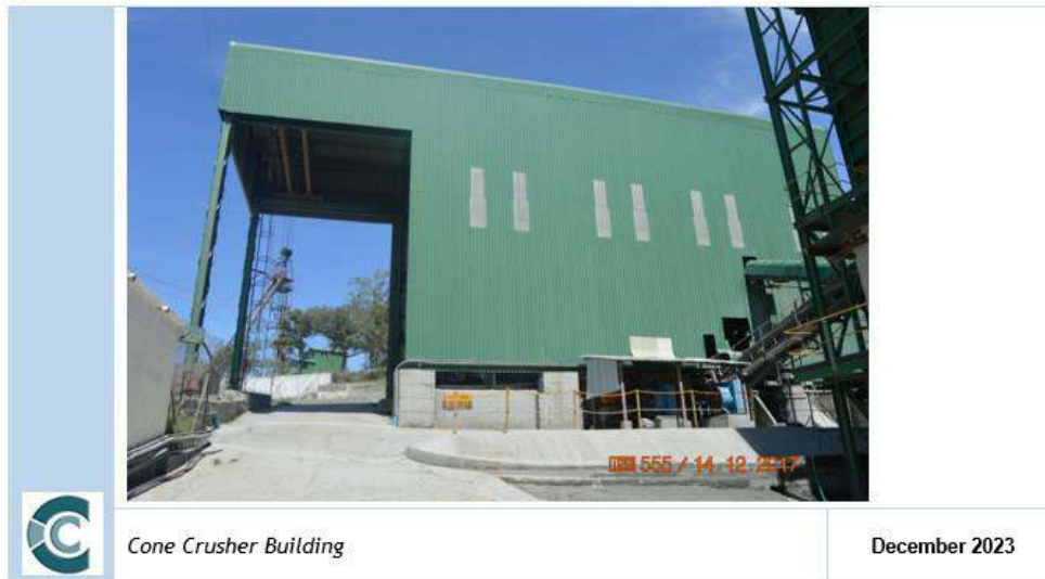
Figure 67: Cone Crusher Building
