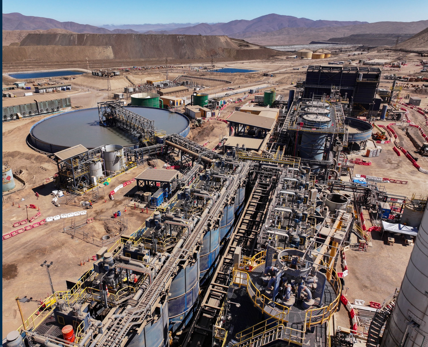
Mantoverde Development Project – March 2024
