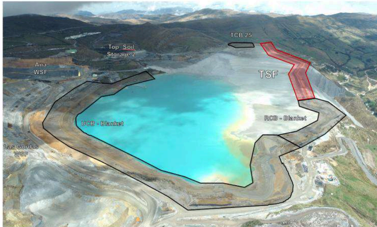
Figure 15.1.2: TSF overview looking west
