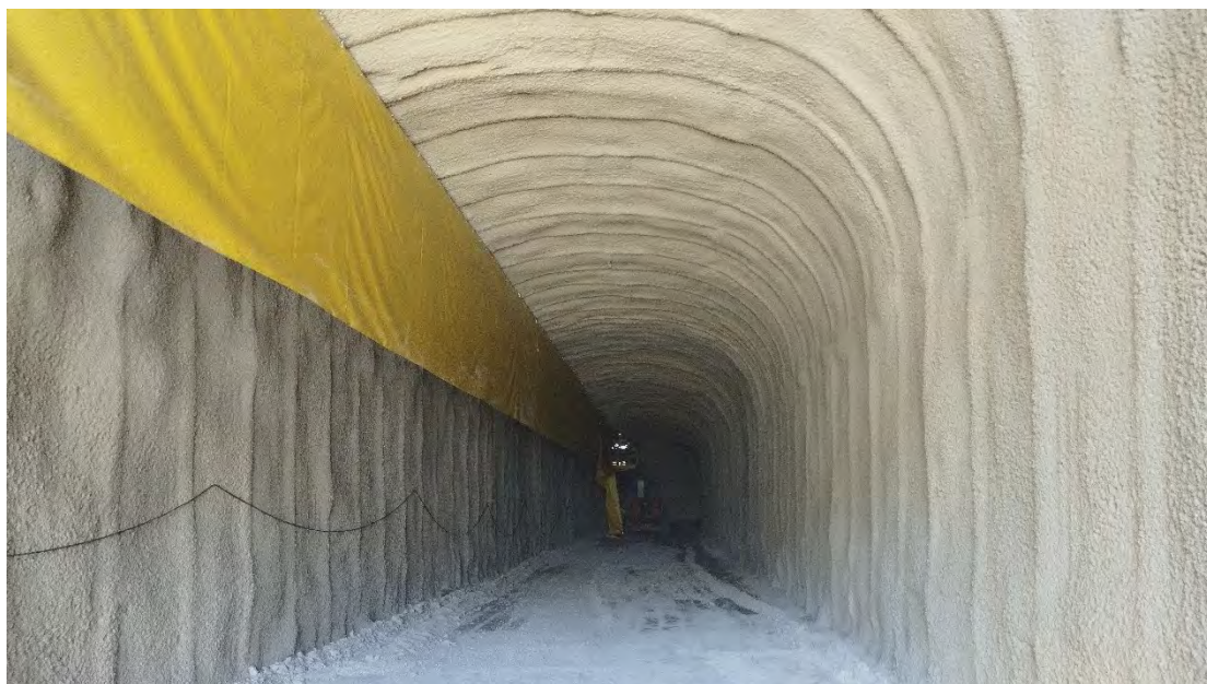
Figure 16-34 Rehabilitation Works at Existing Investigation Ramp
