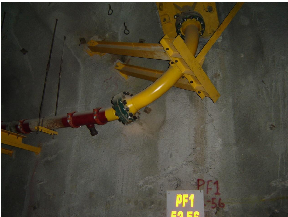
Figure 16.13 – Typical Borehole to Level Piping Connection Configuration
