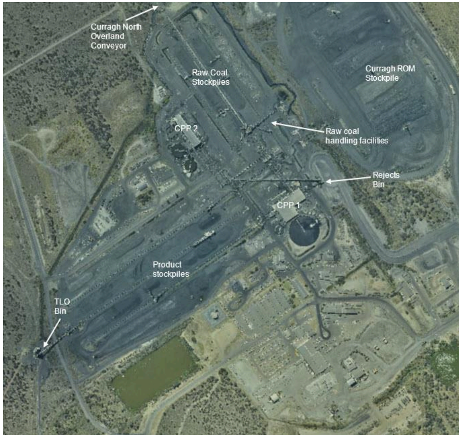
Figure 14-1: Aerial view of the CHPP facilities and associated infrastructure
