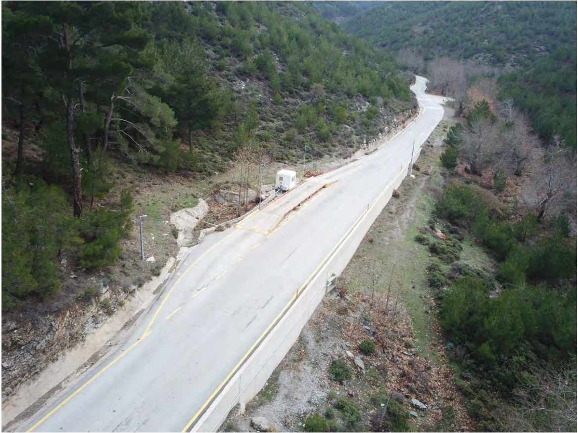
Figure 18-1: Mine Main Access Road
