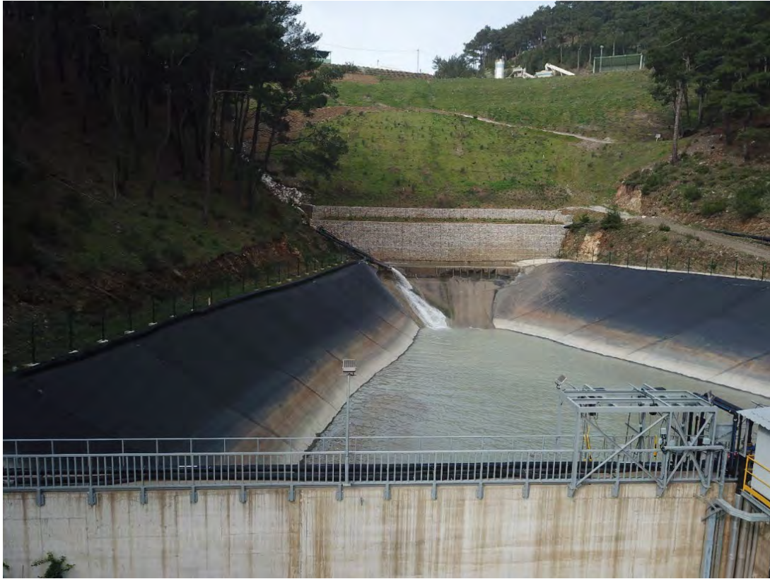
Figure 18-5: Mine Rock Sedimentation Pond (Eldorado, 2019)
