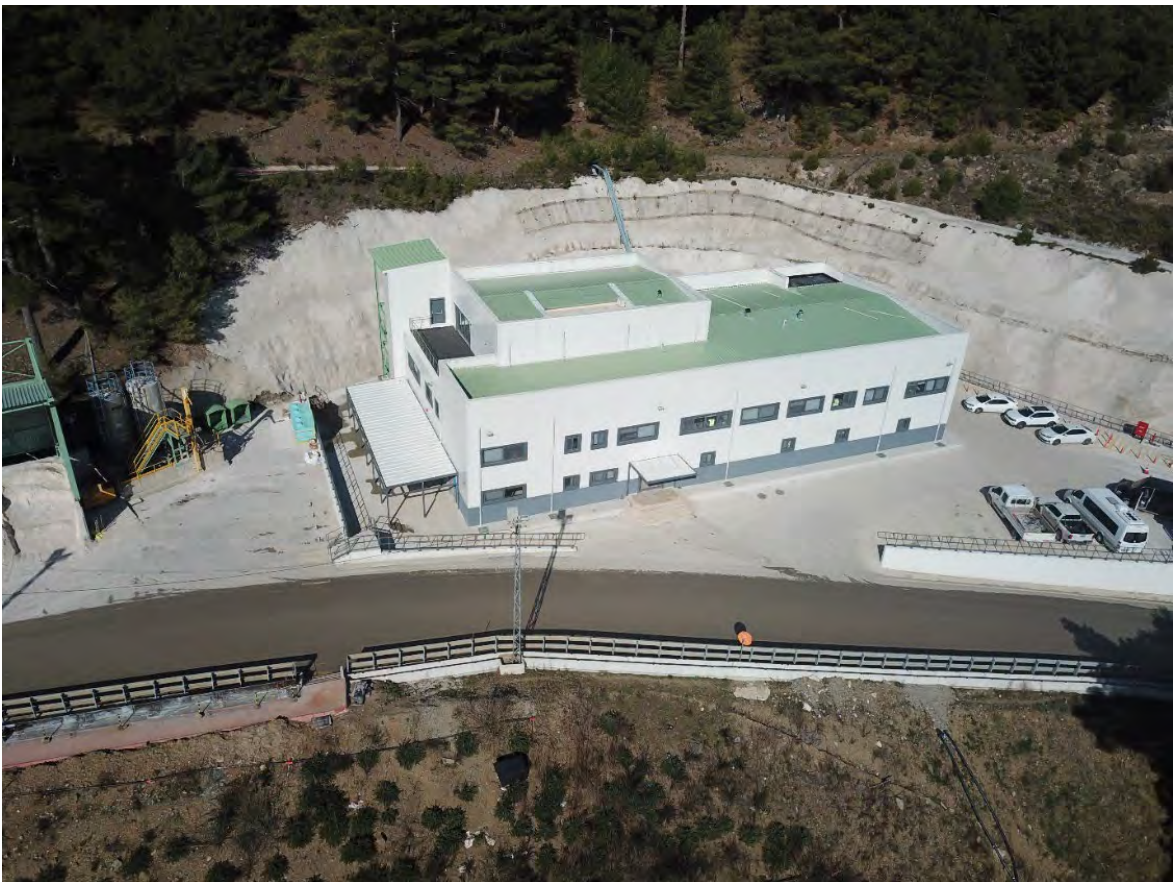
Figure 18-11: Mine Building beside South Portal (Eldorado, 2019)
