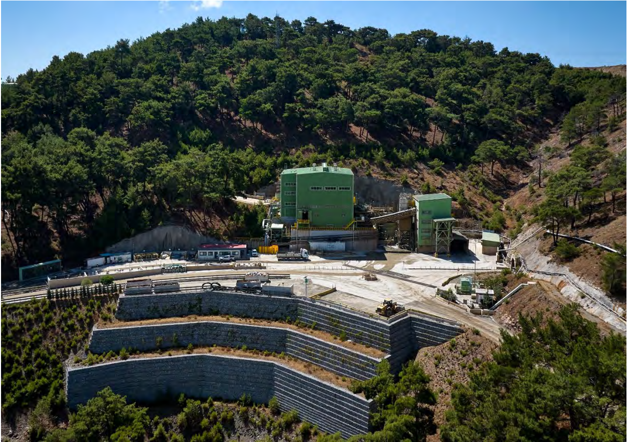
Figure 18-10: Filtration Plant and North Portal (Eldorado, September 2023)
