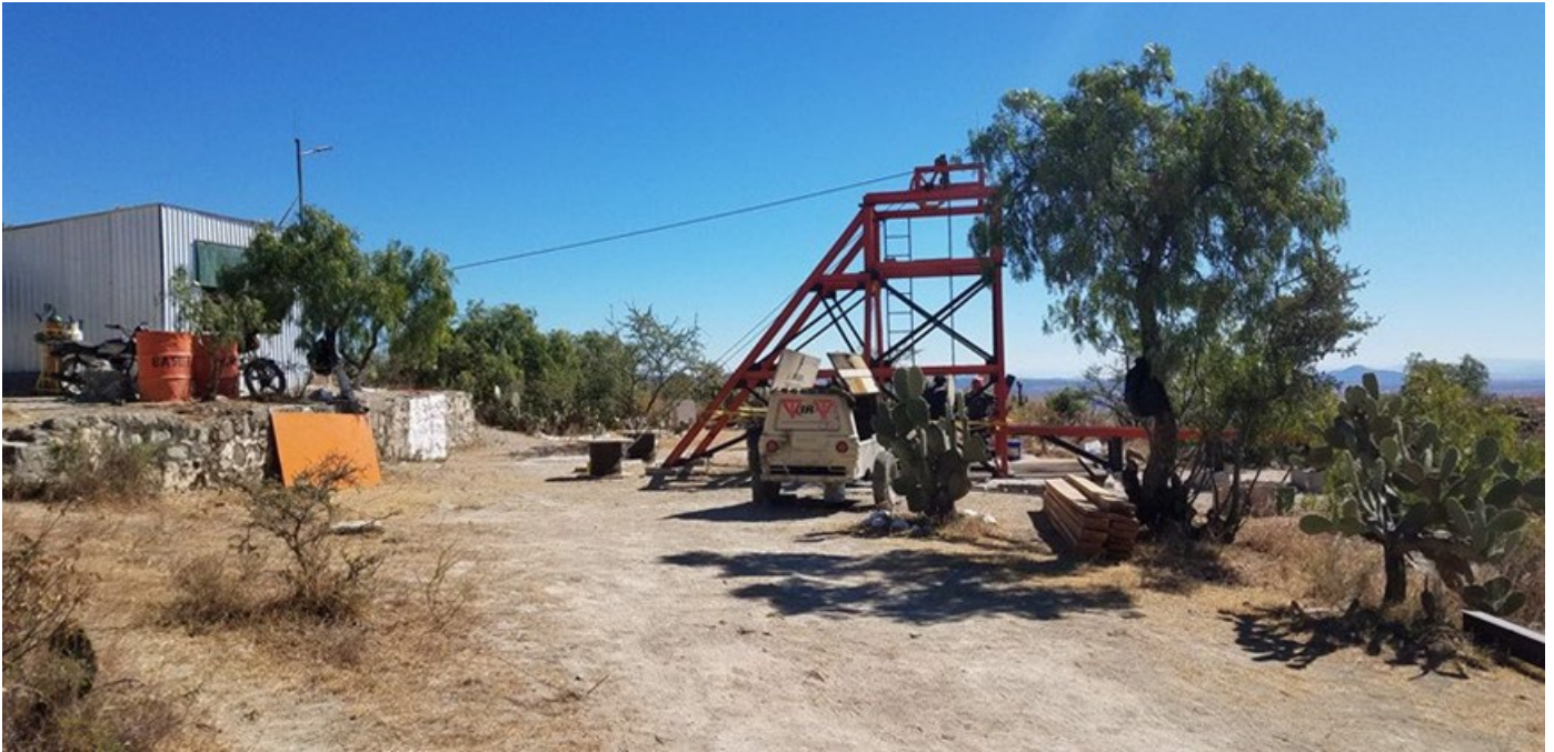
Figure 16.3. El Pingüico shaft Source: Photo taken by John E. Thompson on Site Visit
