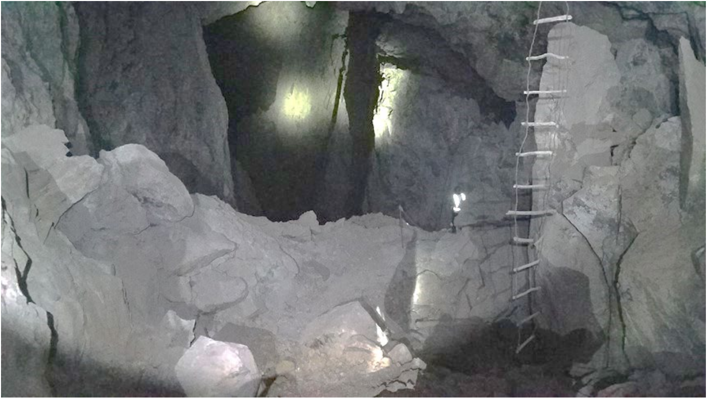
Figure 16.5. Surface of the underground stockpile at Level 4 Source: Photo taken by John E. Thompson on Site Visit
