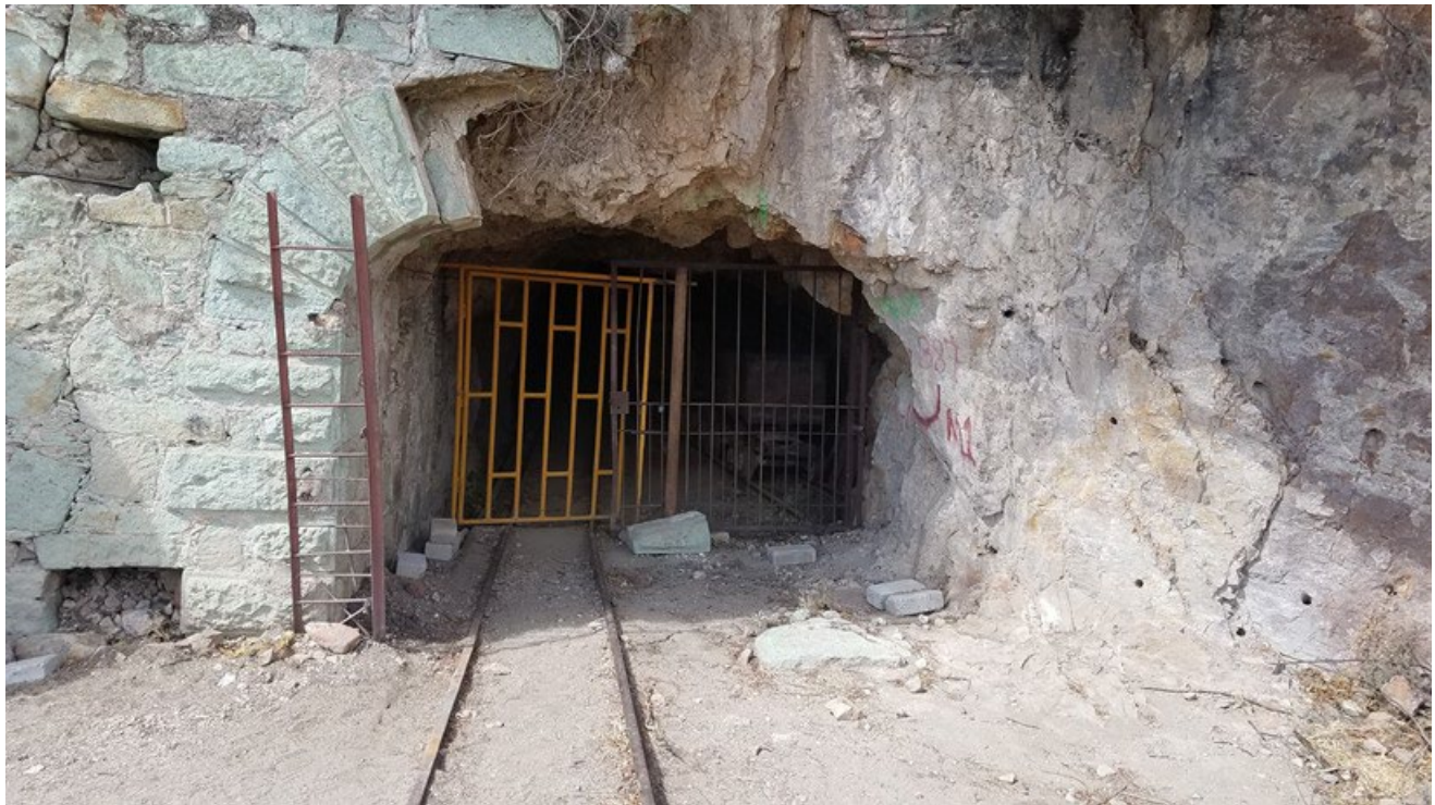
Figure 16.2. El Carmen Portal Level 4 Source: Photo taken by John E. Thompson on Site Visit
