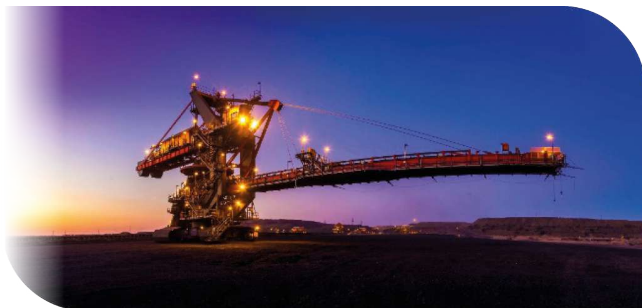
Stacker for discard backfill at Grootegeluk
