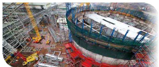
Silo construction at our newly implemented GG6 processing plant
