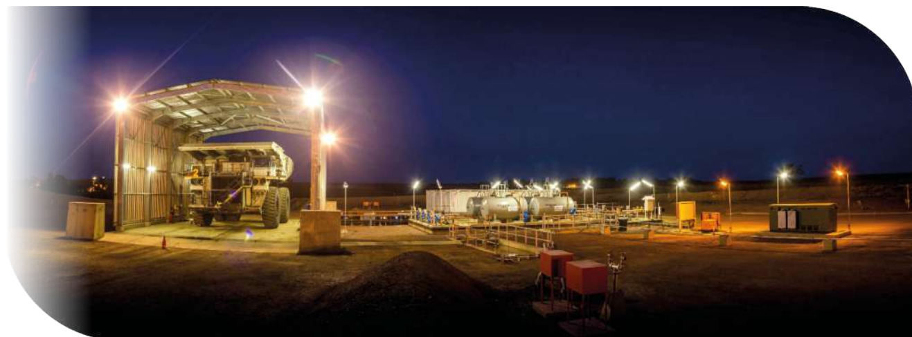
Service bay for production trucks
