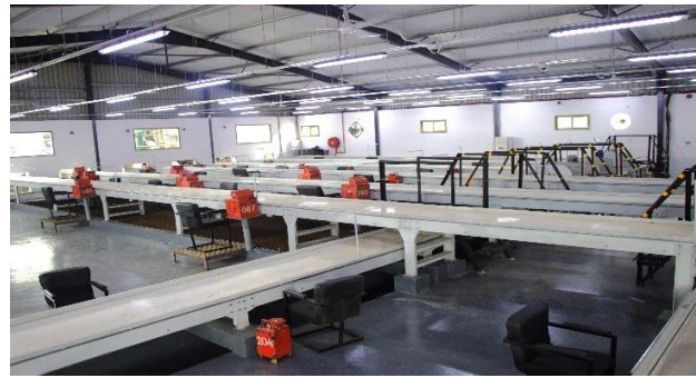
Figure K21: Kagem Wash Plant Rehabilitation of Picking Belt Area
