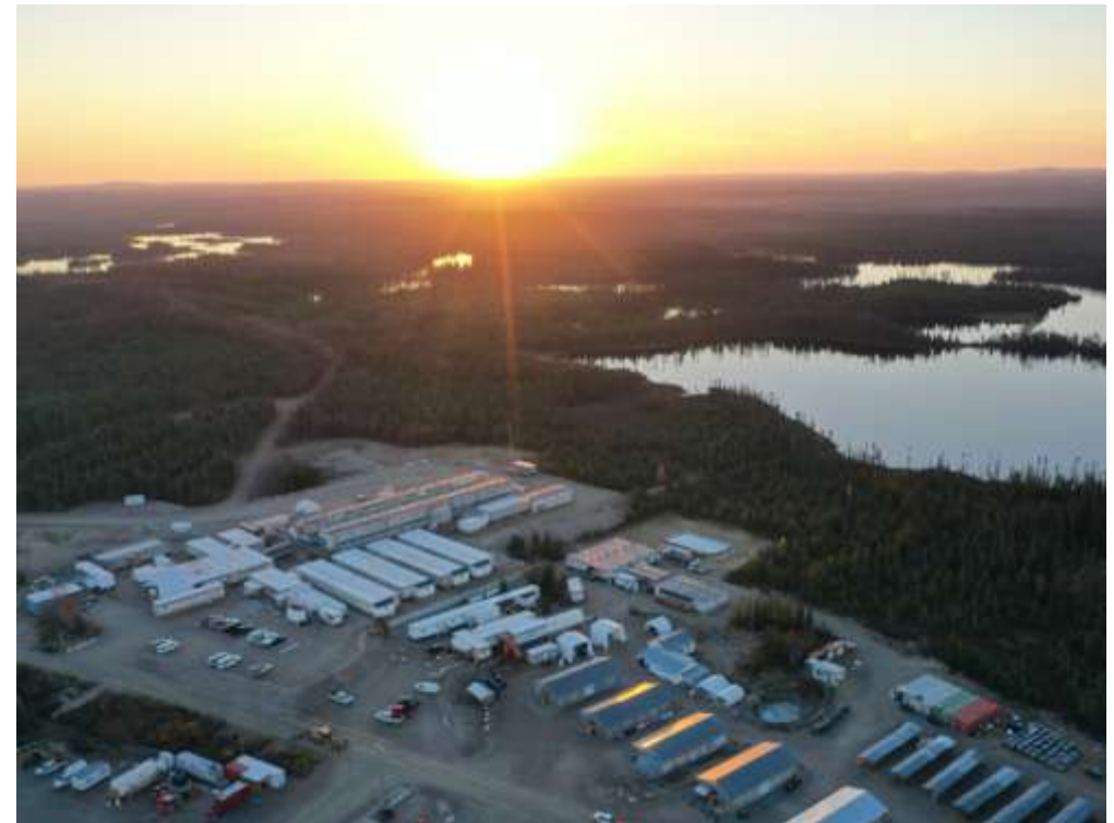
The Windfall project camp and offices in Québec, Canada
