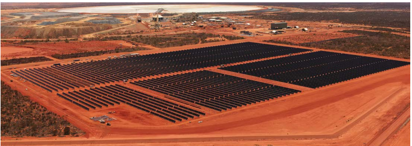
Solar facility at the Gruyere JV gold mine
