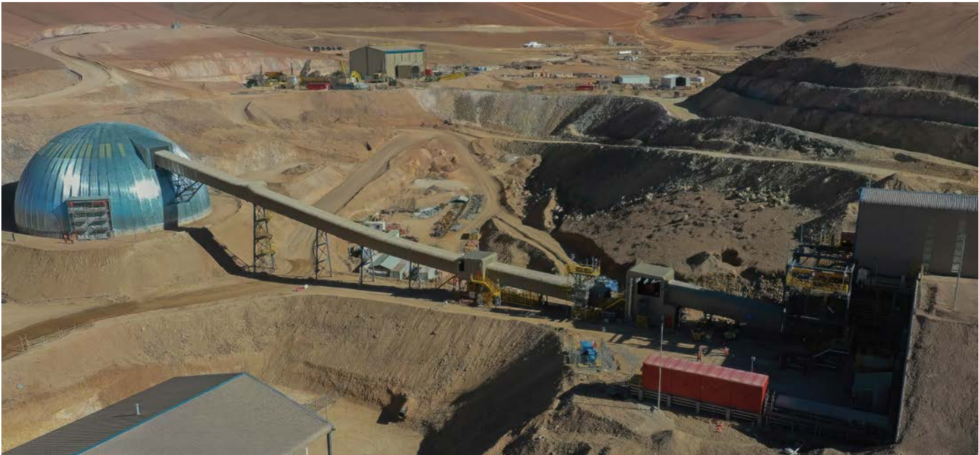
Primary crusher at the Salares Norte gold-silver mine
