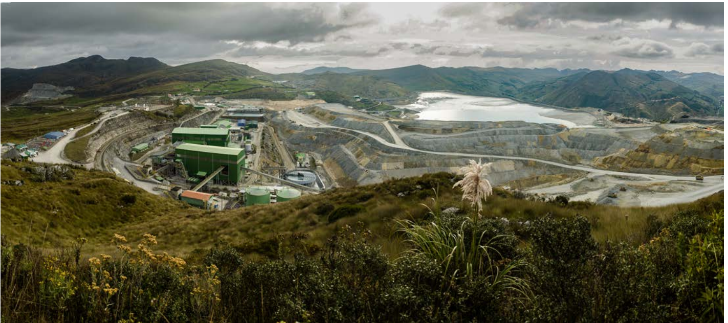
Processing plant at the Cerro Corona gold-copper mine
