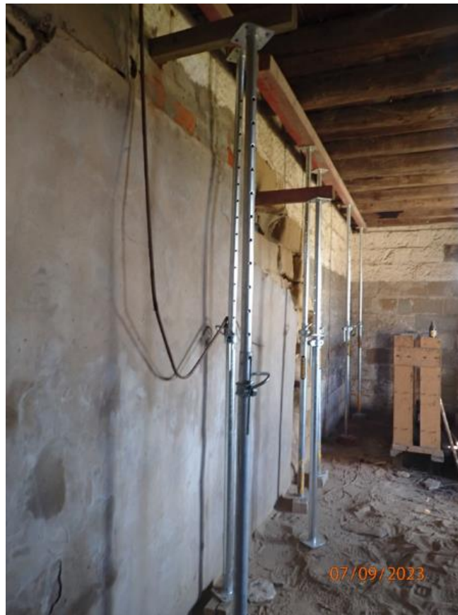
Figure 6-20: Archerfield Homestead Distillery Wall underpinning
