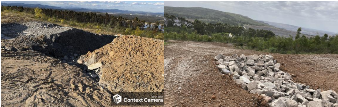
Figure 8-6: Erosion repair at HVOWES202201
