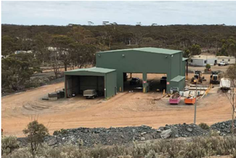
Figure 18-2 HGO underground workshop
