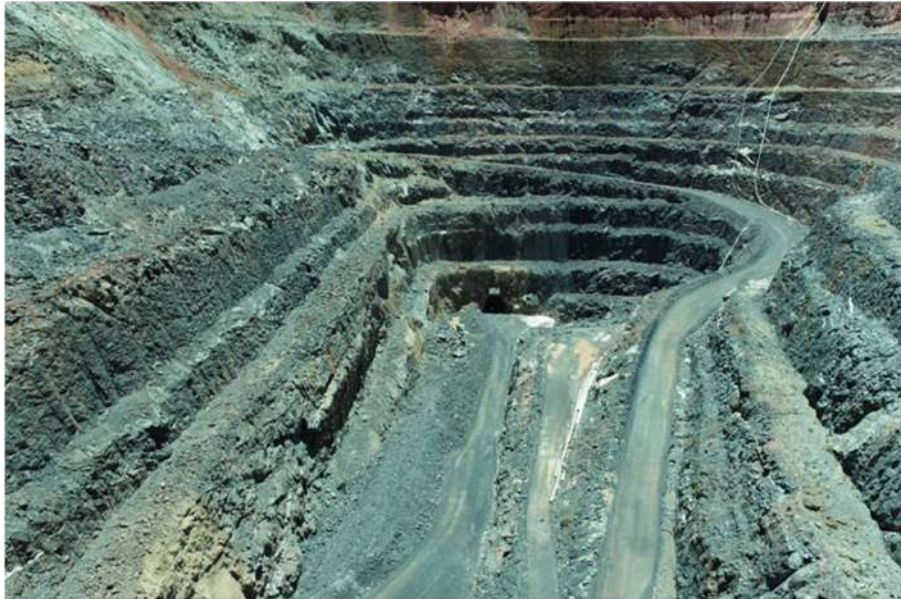
Figure 16-6 Oblique aerial view of Trident Portal inside Poseidon South Pit looking north.
