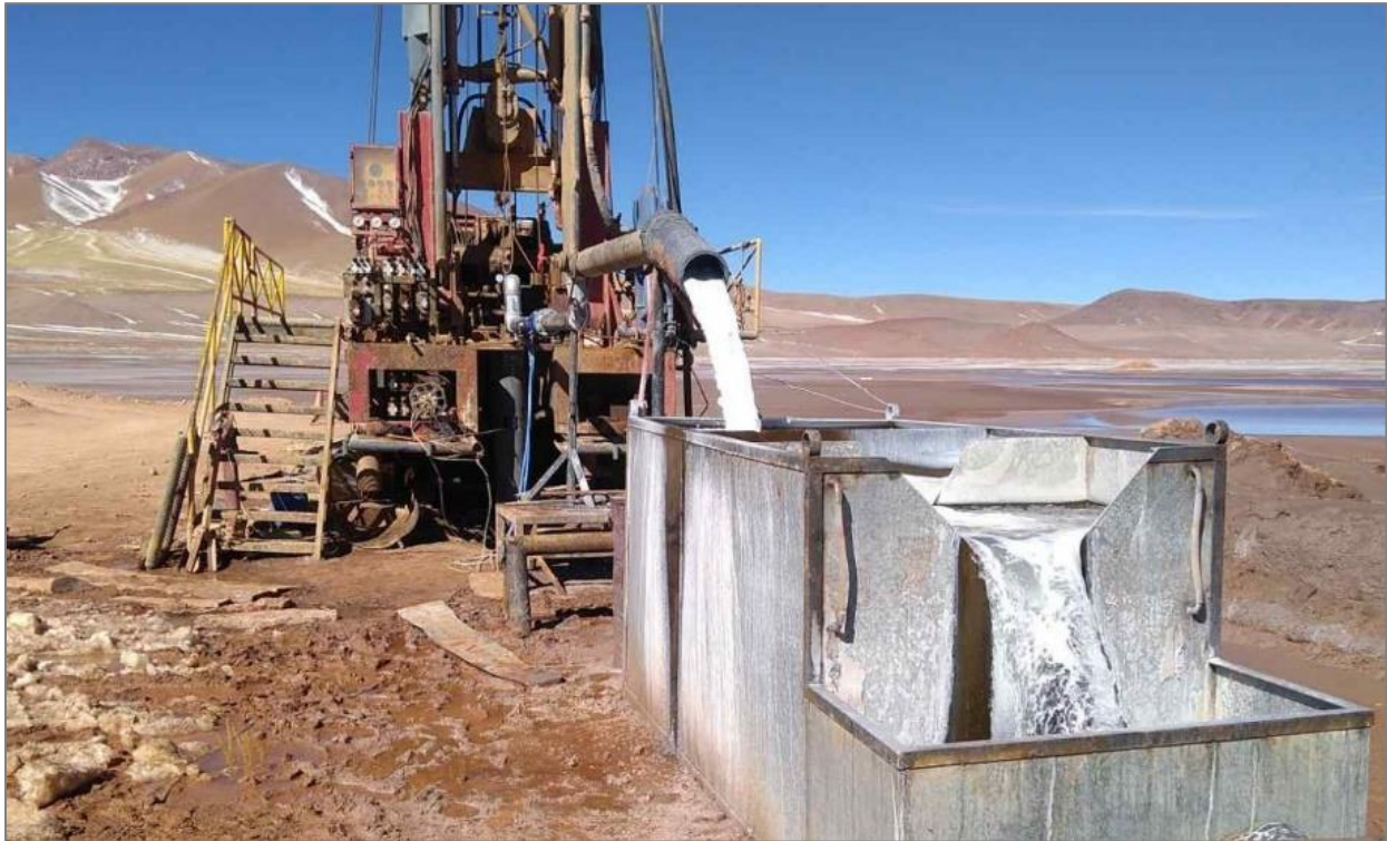
Figure 9-9: 72-hr Constant-Rate Pumping Test Set-up at TWW18-01
