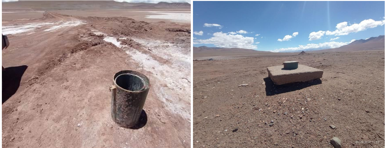
Figure 16-1: Potential Production Wells, Pumping Wells TWW18-01 (left) and TWW18-02 (right), Installed on the Tramo Concessions
