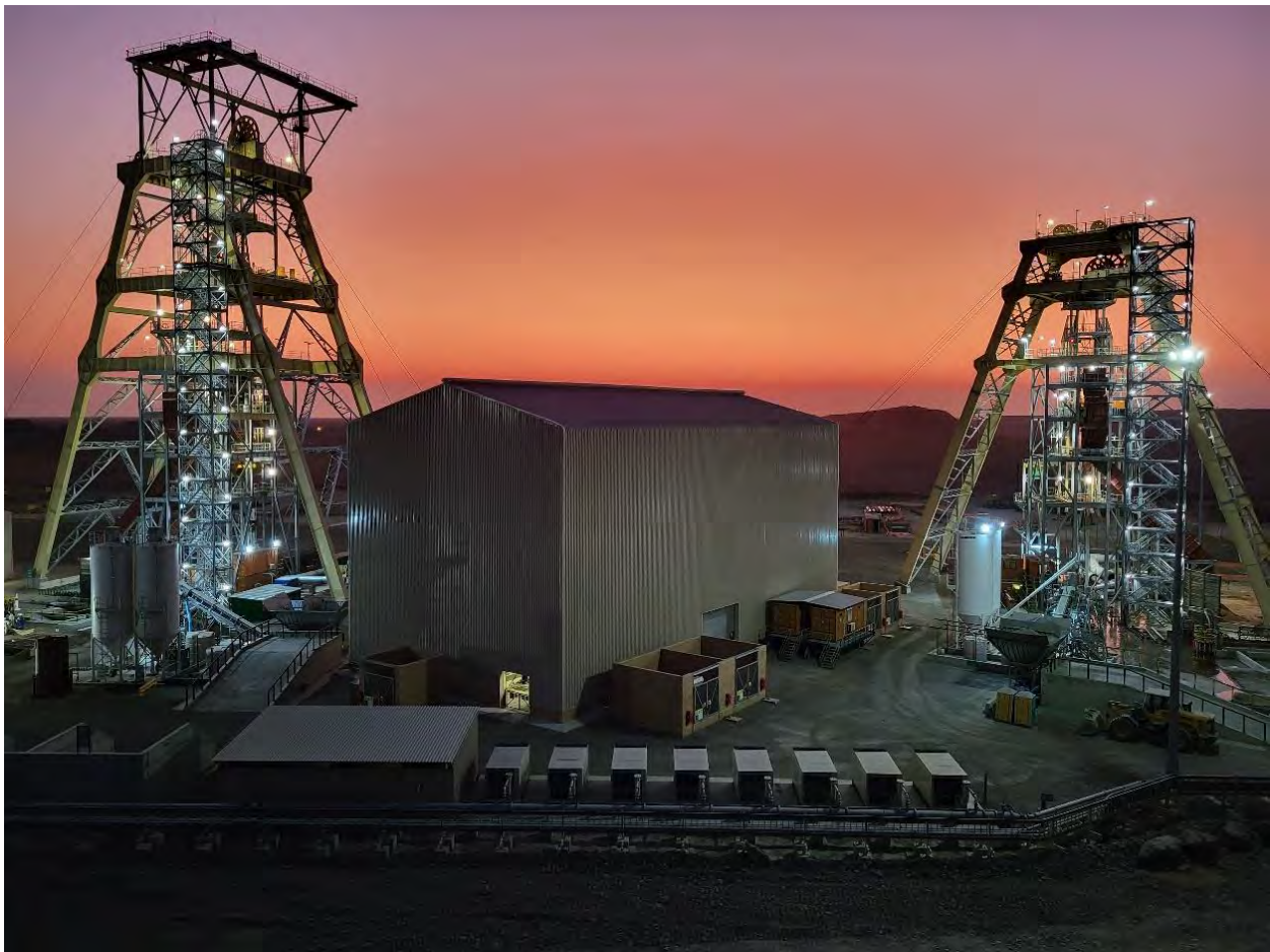
Figure 16-38: Production (left) and Ventilation (right) Shaft Headgear
