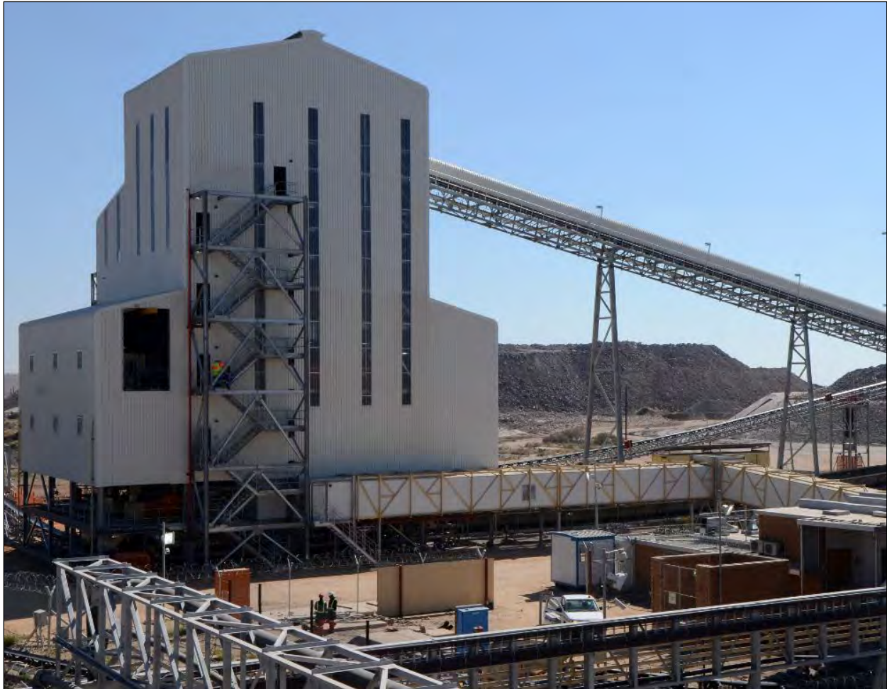
Figure 17-2: Construction Completed and Fully Commissioned KDM Phase II XRT Building
