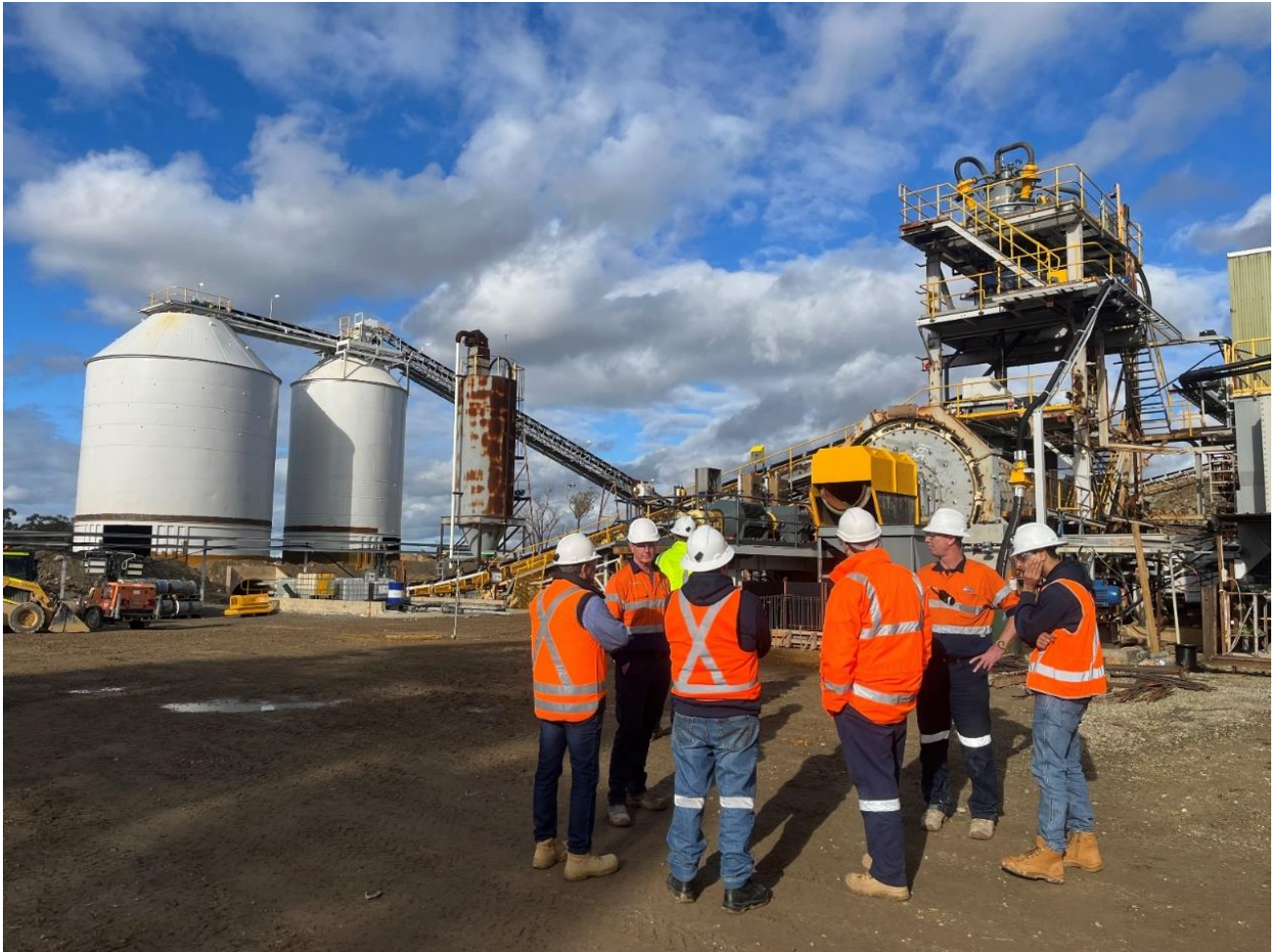
Figure 5: Kingston Board of Directors inspecting the Mineral Hill processing plant commissioning activities.
