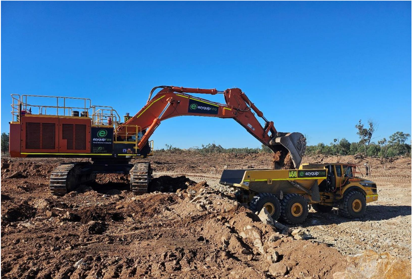
Figure 3: Open pit excavation and haulage.
