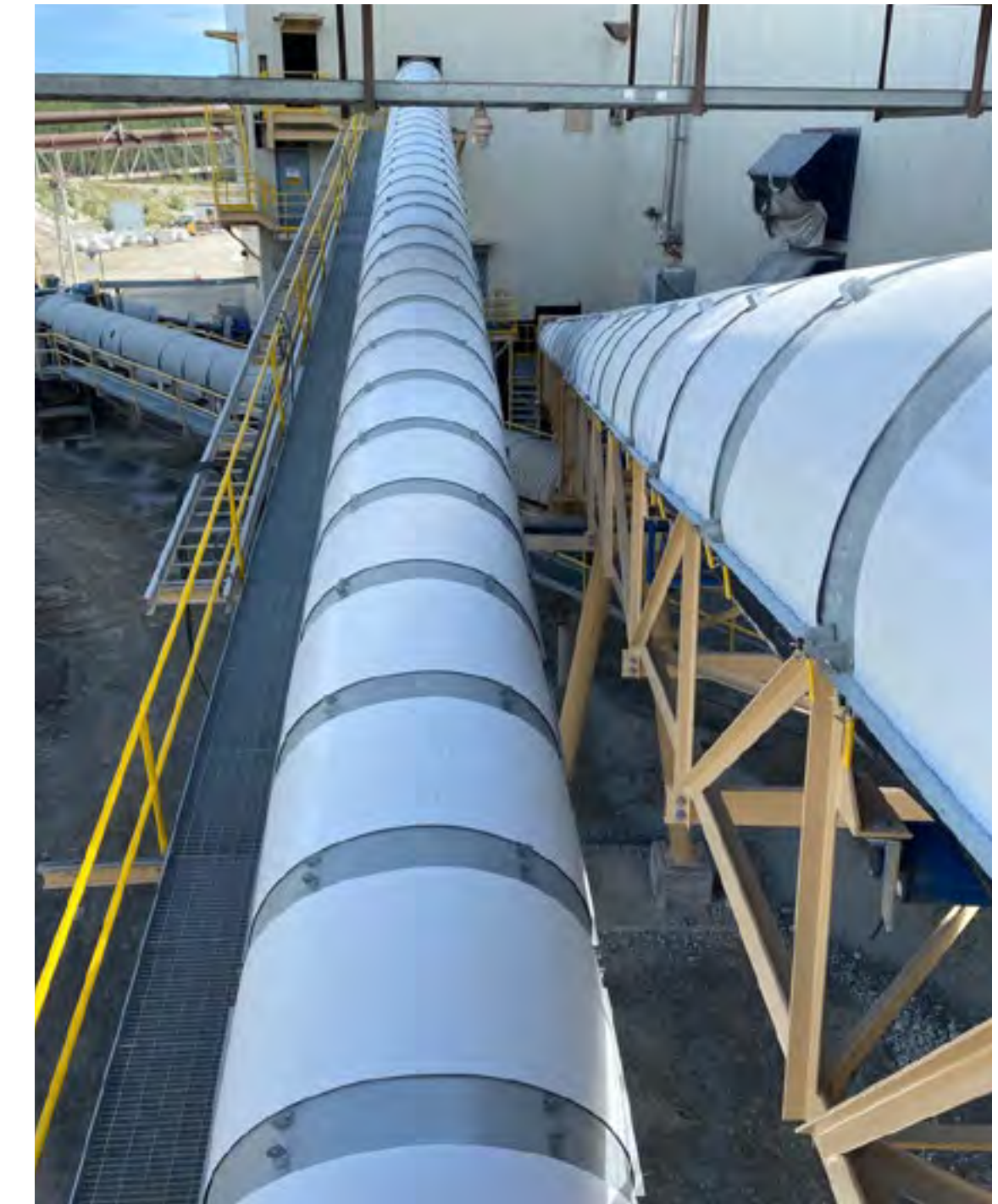
At Fort Knox, a project to reduce the steep incline on a conveyor belt at the mill contributed to load reduction and 2,481,700 kWh in annualized energy savings.
