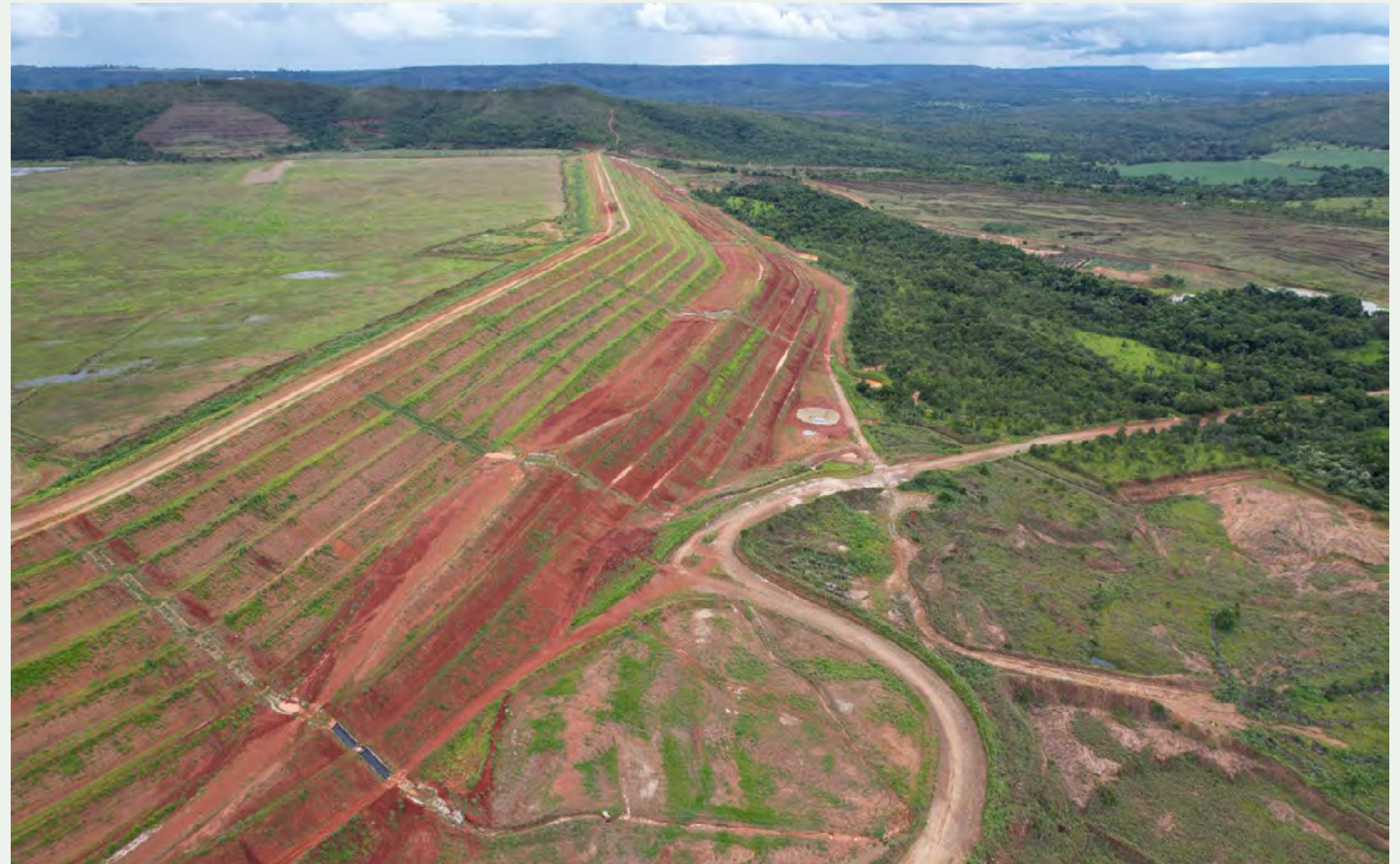
At Paracatu, the closure and reclamation of the Santo Antonio TSF is progressing, with covering and revegetating of the surface, dam face, and borrow areas below the dam.
