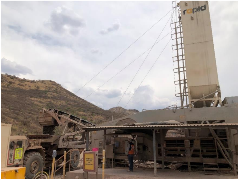
Figure 18.6: CRF Production at the Rapid Mix 400C Plant
