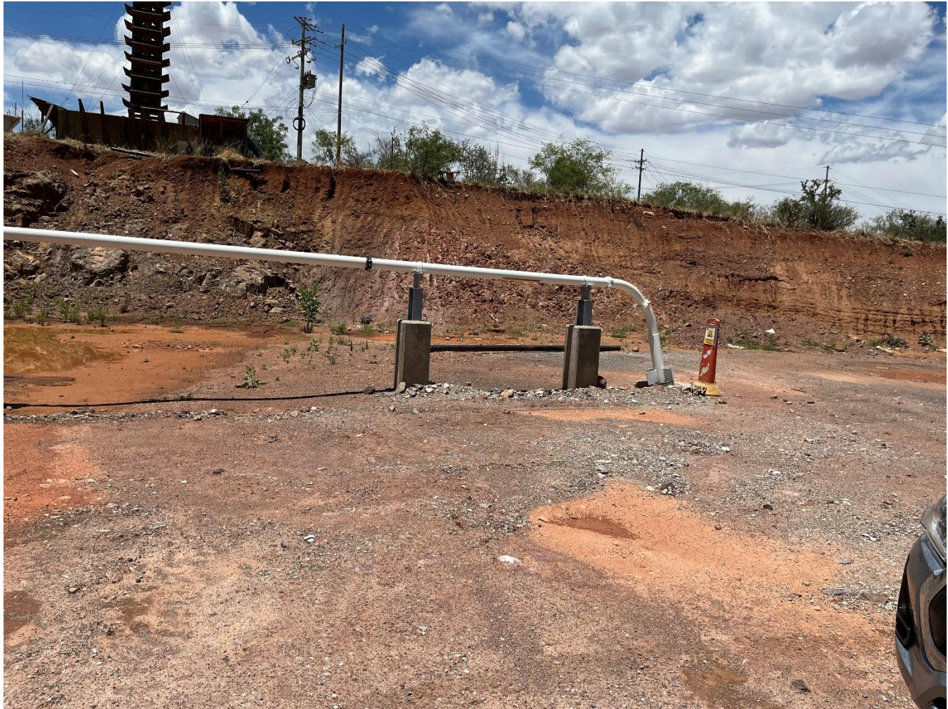
Figure 18.11: Paste Surface Pipeline to Borehole
