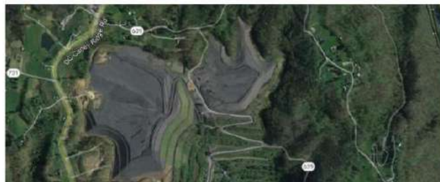
Figure 14-1: McClure River Preparation Plant and Refuse Area
