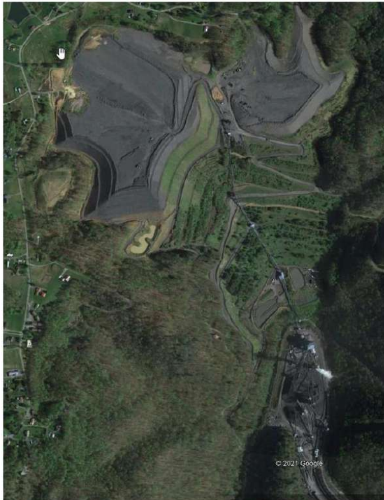
Figure 15-1: McClure River Preparation Plant & Surface Facilities
