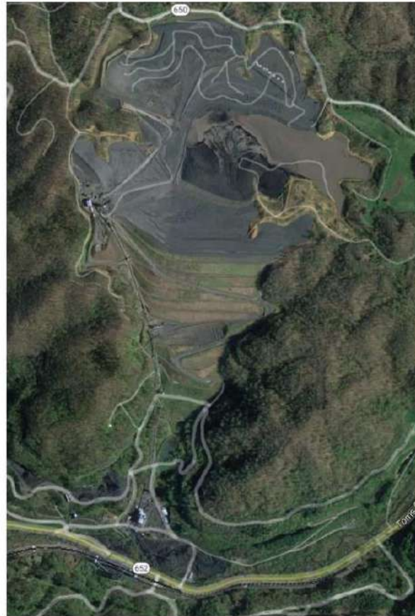
Figure 14-2: Tom's Creek Preparation Plant and Slurry Impoundment
