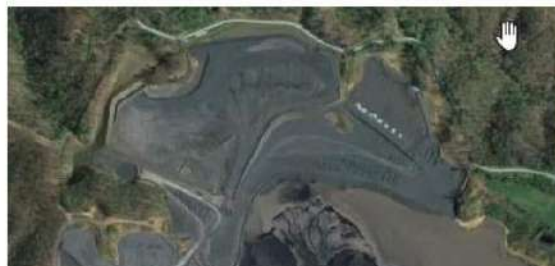
Figure 15-2: Tom's Creek Preparation Plant & Surface Facilities
